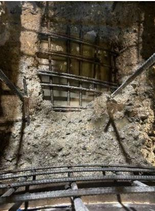
Figure 4.5 – Unit 04 – Non-conforming Concrete
