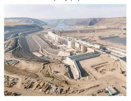
Figure A-10 Riprap is one of the many protective layers in the approach channel where water will flow from the reservoir into the powerhouse and spillways | September 2023
