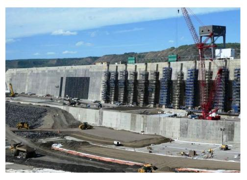
Figure 4.13 – Intakes and RCC Tailrace Wall
