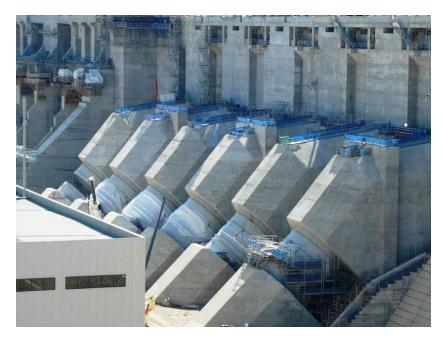
Figure 5.1 – Penstock Flexible Joints
