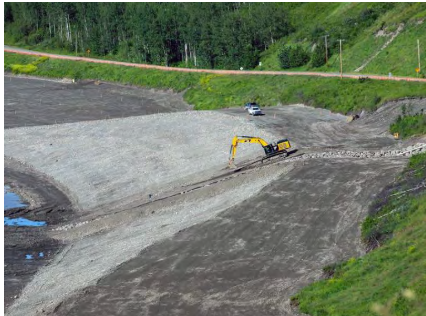
Figure A-26 Roadway embankment construction upstream of Dry Creek (July 2020)
