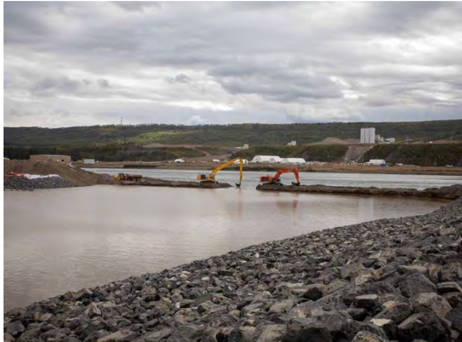
Figure A-37 Removing the inlet portal cofferdam (September 2020)
