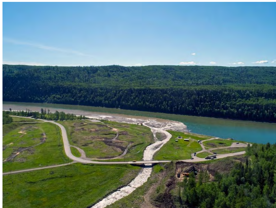
Figure A-20 Highway 29 realignment work at Lynx Creek (June 2020)
