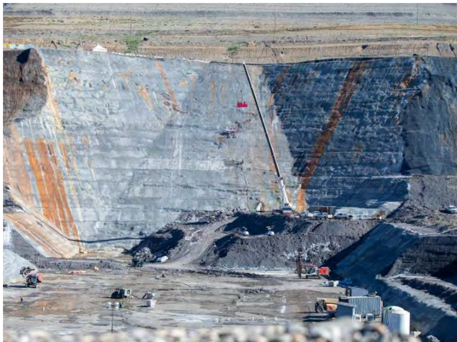
Figure A-38 Overview of the left bank core trench excavation (September 2020)
