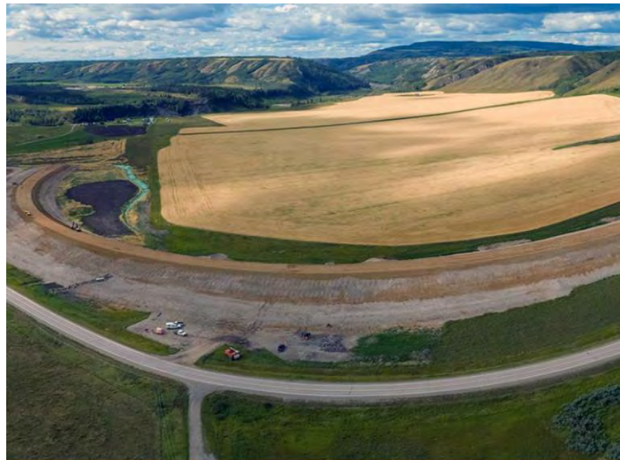
Figure A-32 The completed Cache Creek East embankment on Highway 29 (August 2020)
