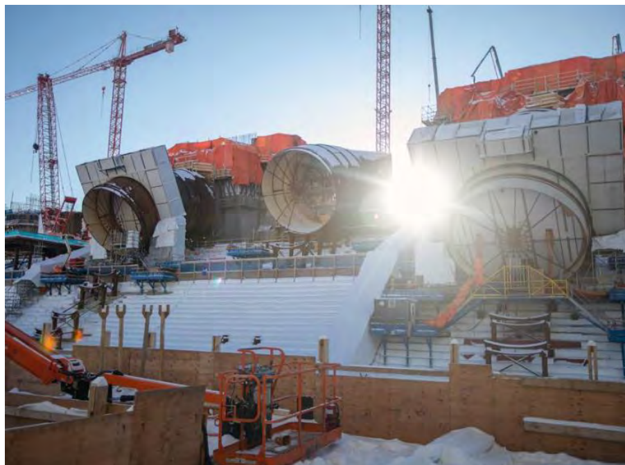
Figure A-2 Penstock construction of units 1, 2 and 3 (January 2020)
