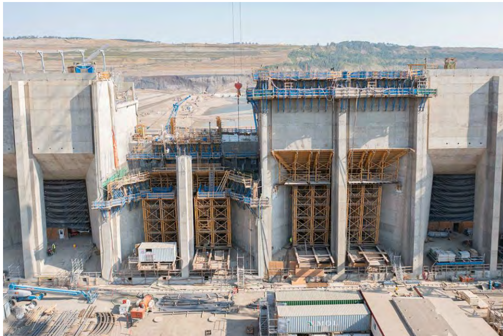
Figure A-10 Construction of the intake gates for units 4 and 5 | August 2022
