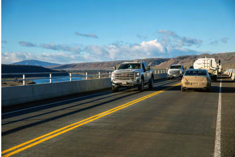
Figure A-21 Farrell Creek Bridge open to traffic on October 27 | October 2022
