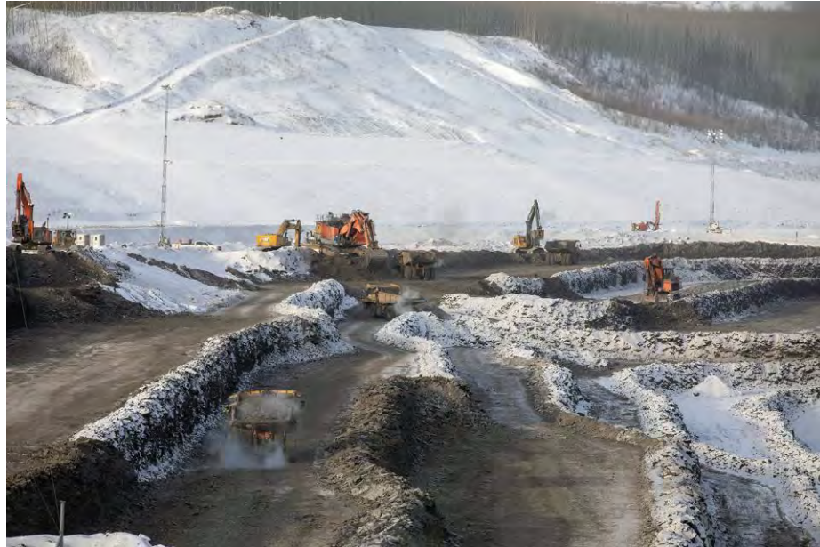
Figure A-1 Excavation work continues at the approach channel | January 2022
