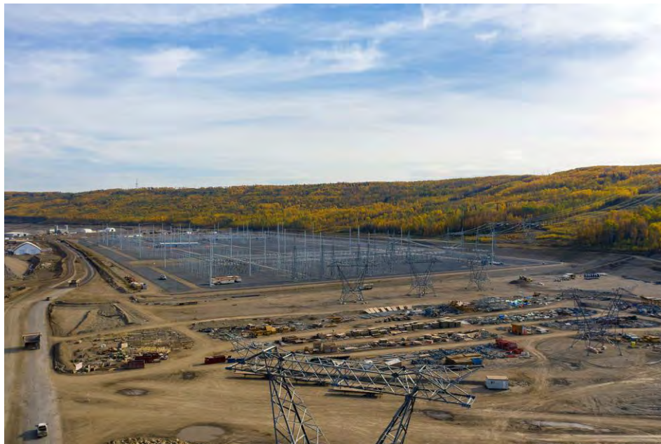
Figure A-12 East-facing view of the completed Site C substation. Transmission lines will be installed on the towers in the foreground to connect the substation to the Site C dam and generating station | September 2022
