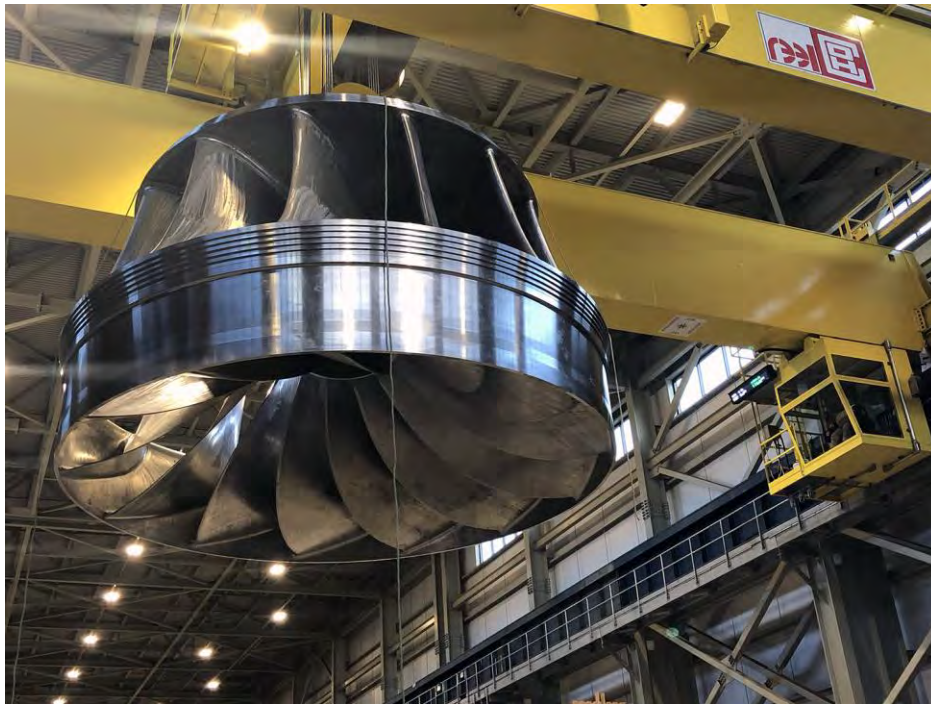
Figure A-22 Installation of the unit 1 turbine runner | October 2022
