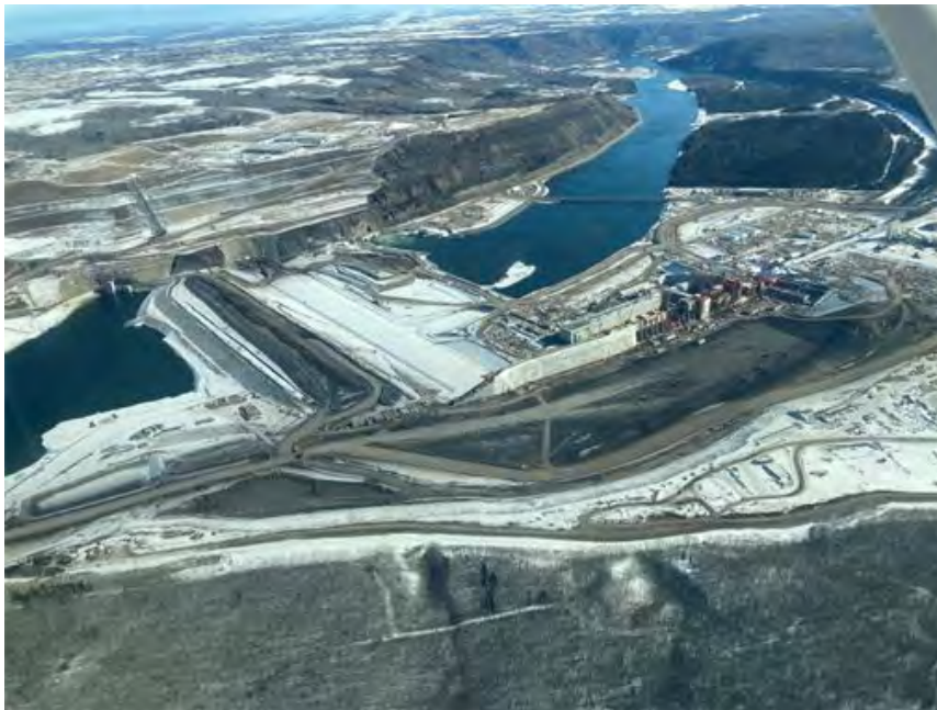
Progress Photo, March 2022
