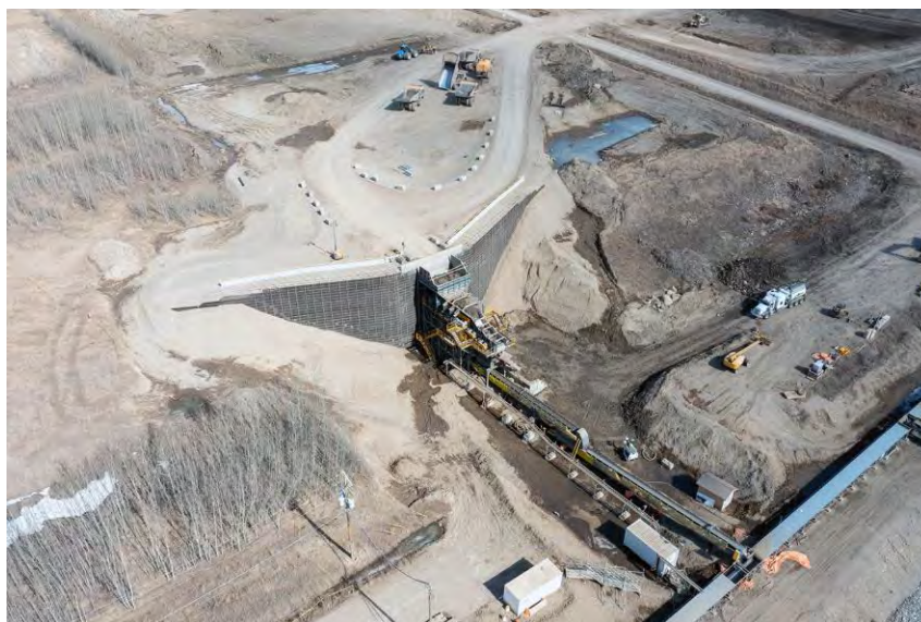
Figure A-6 The hopper and feeder are the primary supply loading point for the conveyor that transports glacial till from the 85th Ave Industrial Lands to Site C | April 2022
