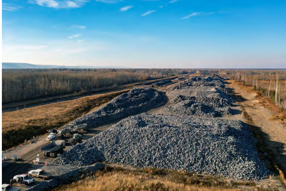
Figure A-15 Riprap stockpile at Septimus rail siding | October 2022
