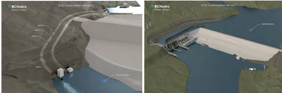
Figure 3. The image on the left shows the start of reservoir filling with water flowing through the converted Tunnel 2 after the closure of Tunnel 1 at El. 425 m. The image on the right shows flow of water into the Approach Channel.
