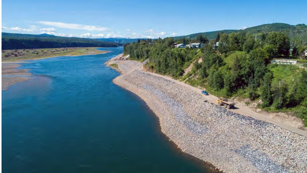
Figure A-9 Progress on the Hudson’s Hope shoreline protection berm | July 2022
