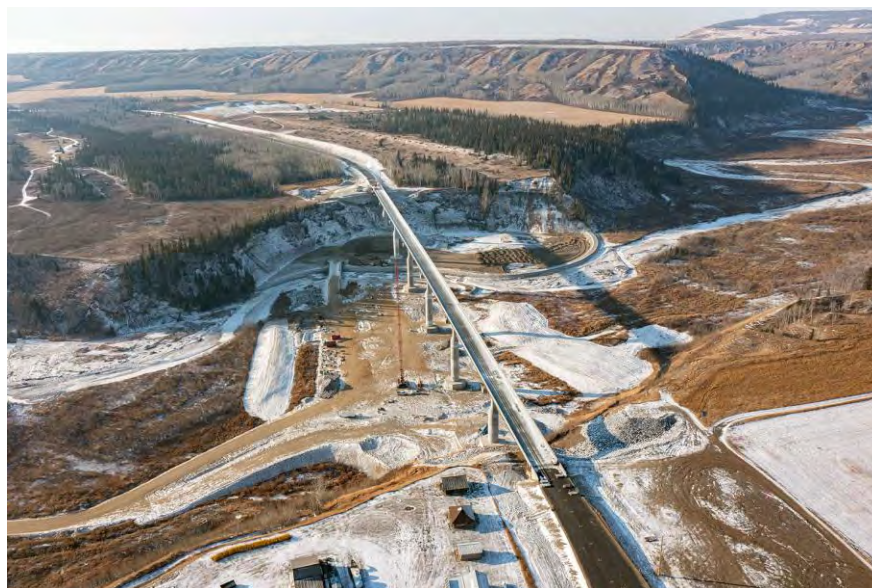
Figure A-26 Completed Cache Creek Bridge on Highway 29 | November 2022
