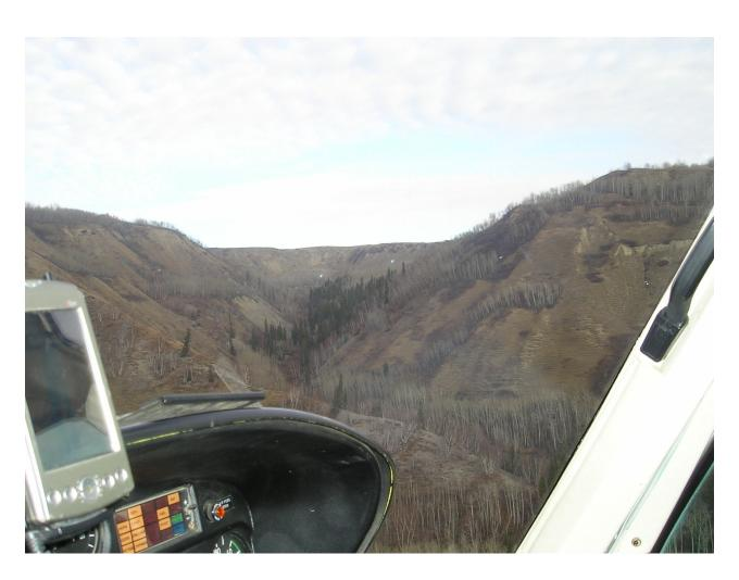
Site C2 – Hovering over the right bank looking across on the dam axis. Note the slides over the left abutment.
