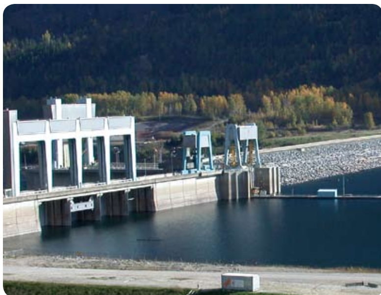
Hugh Keenleyside Dam, near Castlegar.
