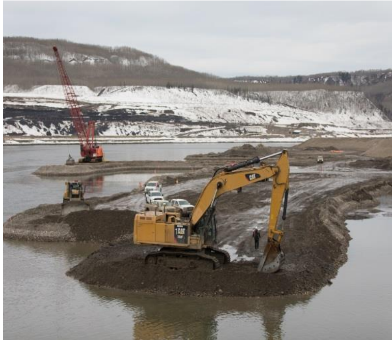
Figure A-3 In-river Works (Dredging). Photo taken April 19, 2018.
