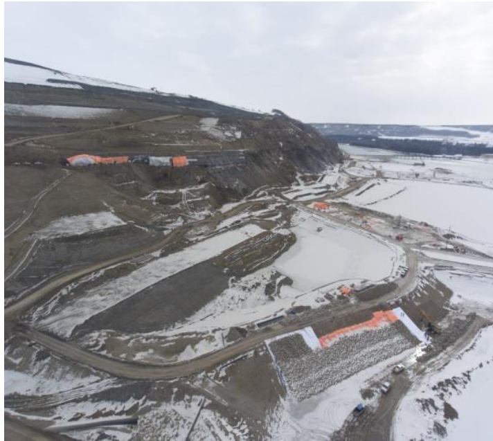
Figure A-1 Left Bank Cofferdam. Photo taken April 5, 2018.
