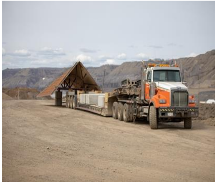
Figure A-5 Transition segment for Unit 1 of 6 of the penstocks. Each penstock starts with a transition piece that is shipped in four parts, each weighing 13,243 kilograms or 31,400 lbs. (April 2019).
