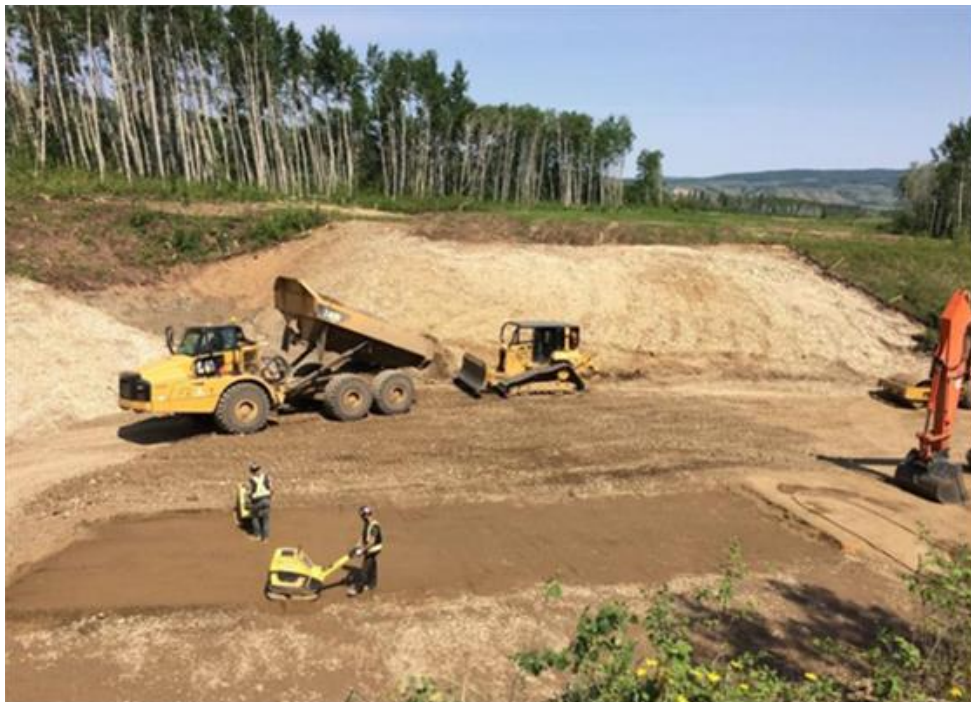
Figure A-8 Grading and levelling is occurring on the new alignment of Highway 29 at Cache Creek West (June 2019).
