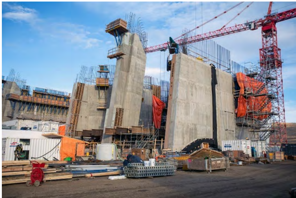
Figure A-38 Construction of the intake gate of penstock Unit 3 (November 2019)
