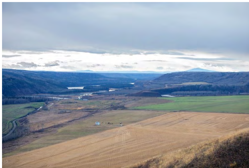
Figure A-26 The Halfway River Segment of the Highway 29 Road Alignment is Four-km Long, Including a One-km-Long Bridge. Preparation Work Began in 2019 and Completion is Scheduled for 2022 (October 2019)
