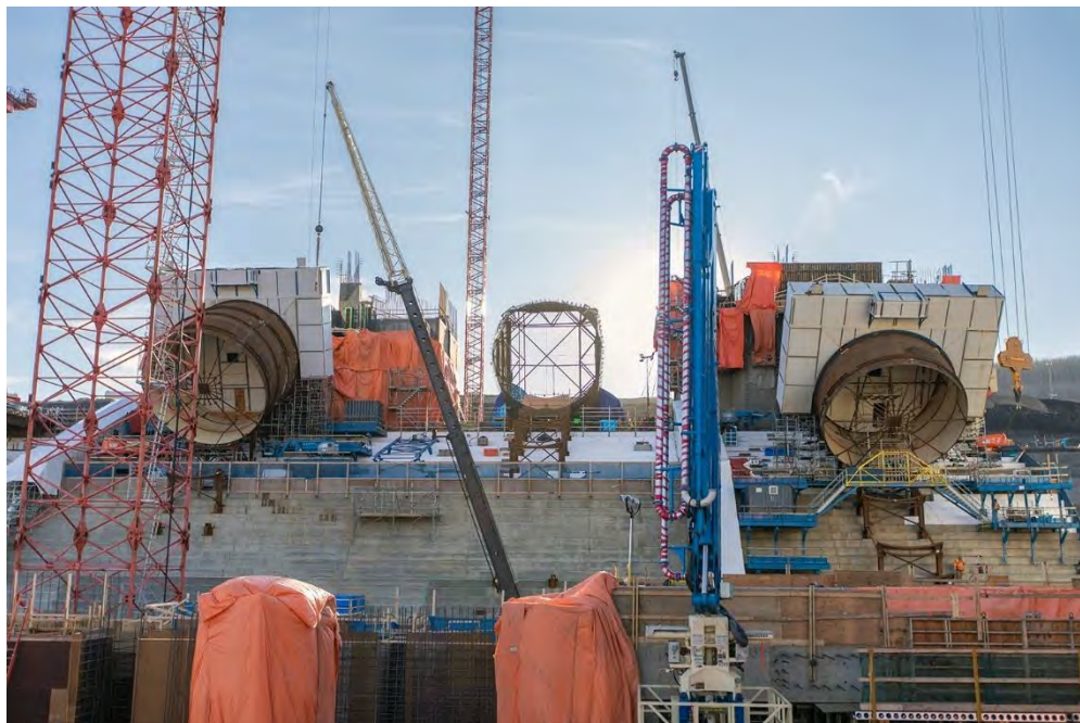
Figure A-30 Penstock Units 1, 2 and 3 in Varying Stages of Construction (October 2019)
