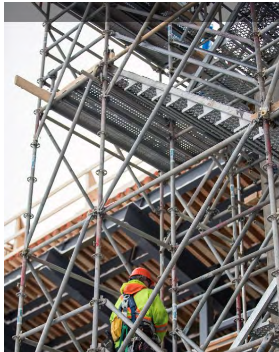
Figure A-4 Inspector Reviewing and Certifying that Scaffolding is Safe and Complies with Regulations. All parts of the Project are Regularly Monitored by Environmental and Safety Inspectors (January 2019)
