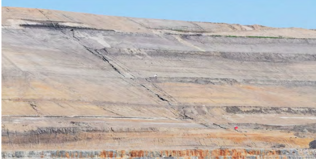
Figure 3: Gullying in unprotected glacio-lacustrine soils of left bank slope
