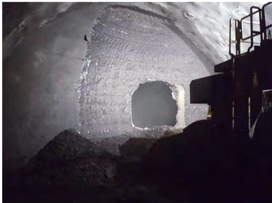
Figure A-16 Diversion Tunnel No. 2 Breakthrough (July 2019)
