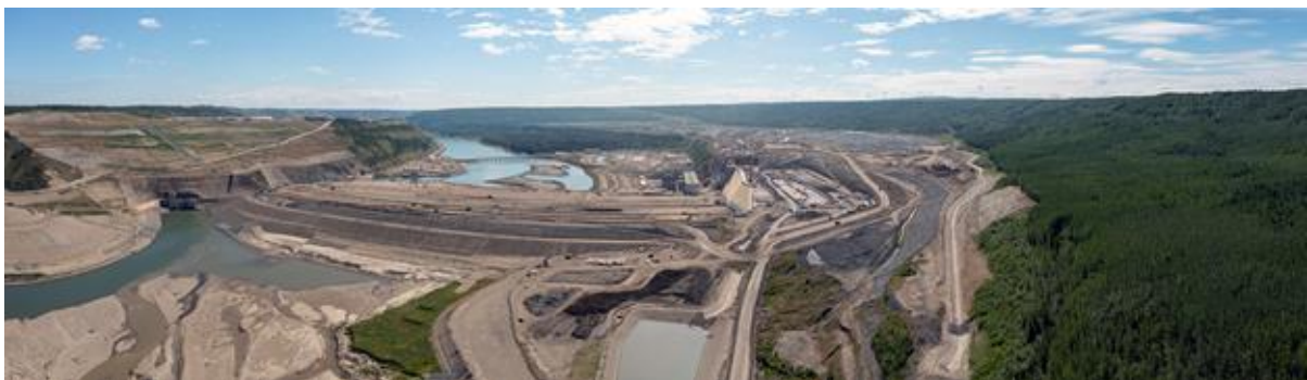
Figure A-4 Panorama view, looking downstream, over the diversion tunnel inlet portals on the left, the earthfill dam in the centre, and the approach channel on the right (July 2022)
