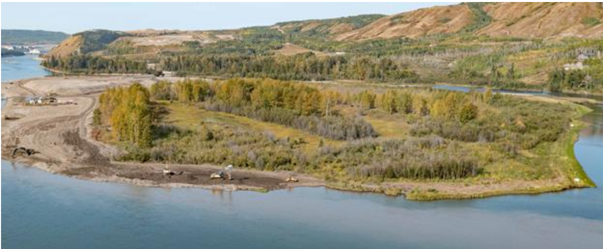
Figure A-8 Fish habitat enhancements downstream of the dam site (September 2022)
