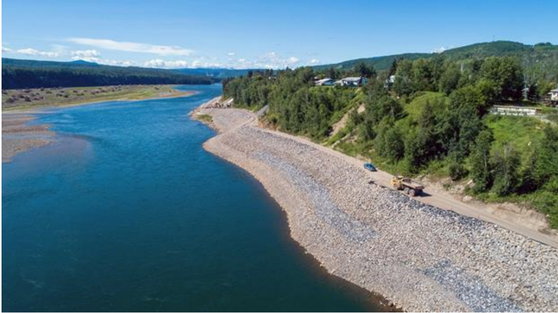
Figure A-1 Progress on the Hudson’s Hope shoreline protection berm (July 2022)
