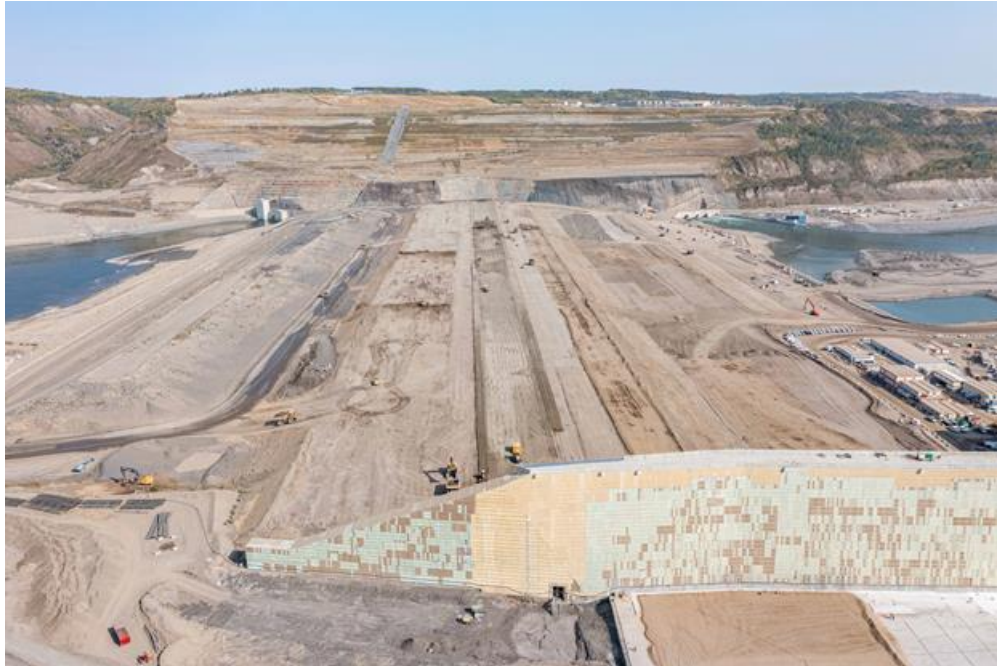
Figure A-7 The Site C dam under construction, looking north (September 2022)
