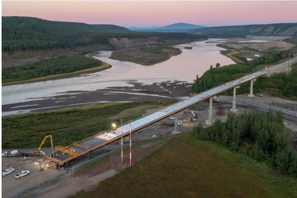
Figure A-5 Farrell Creek final concrete placement (August 2022)
