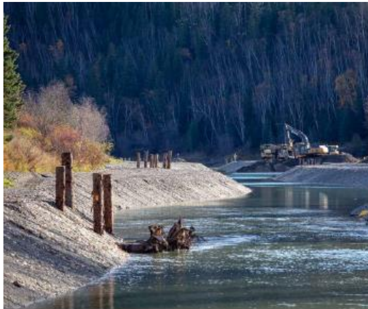
Construction of new downstream channels for fish habitat
