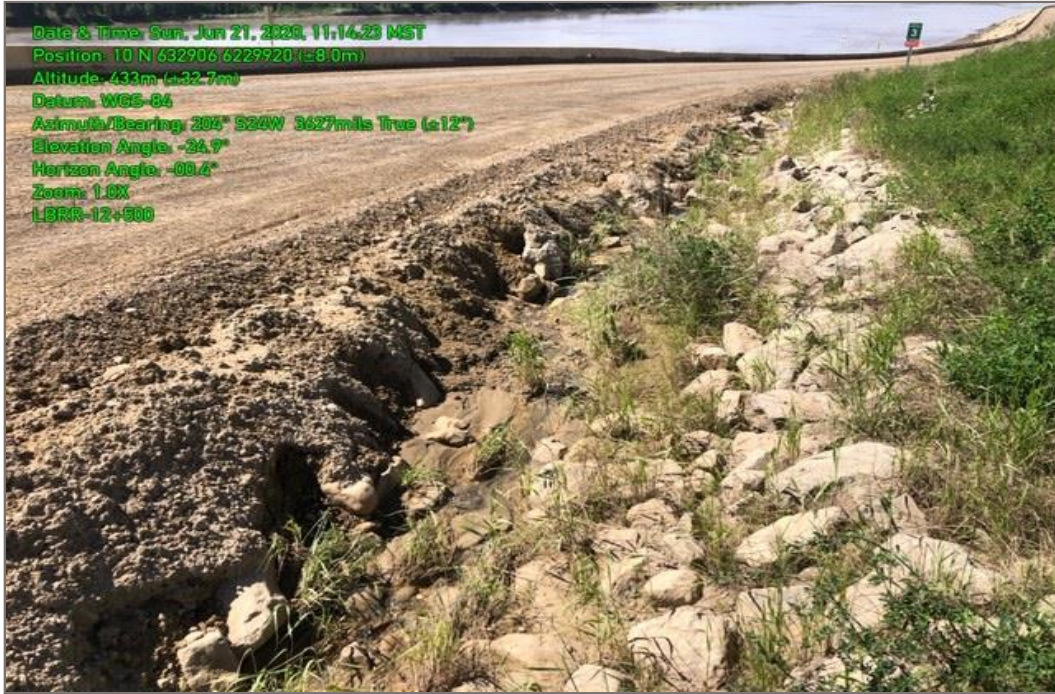
Photo 5: River Road LBRR-12+500 location, June 21, 2020.
