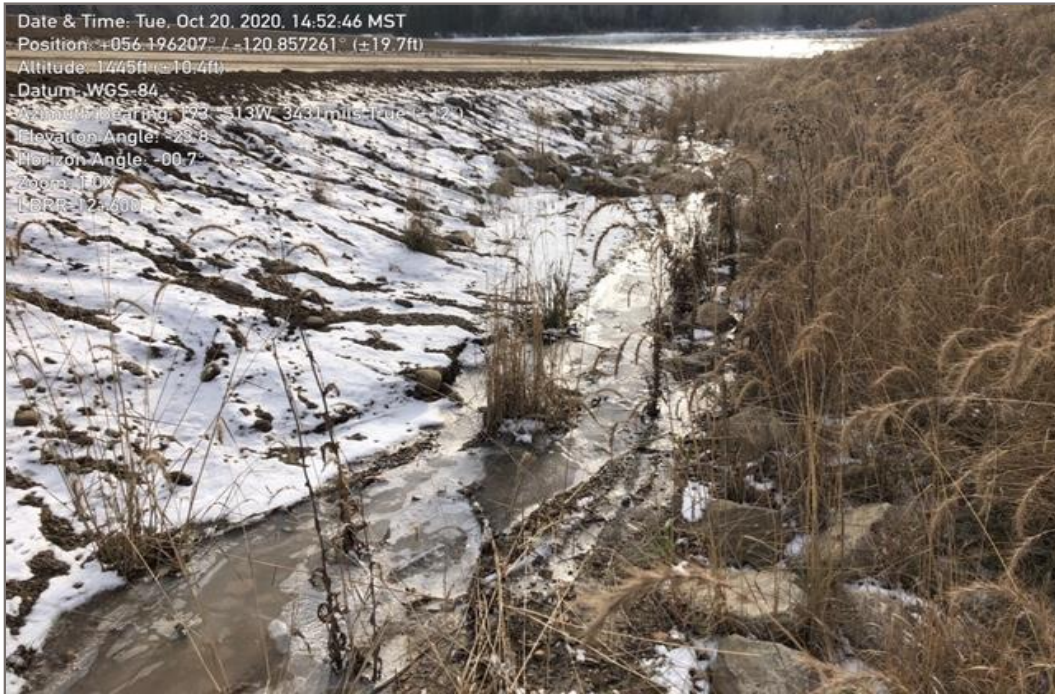
Photo 6: River Road LBRR-12+600 location, October 20, 2020.
