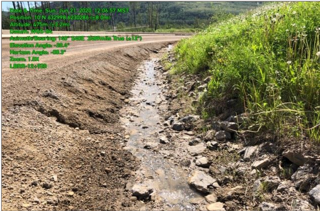
Photo 9: River Road LBRR-12+920 location, June 21, 2020.
