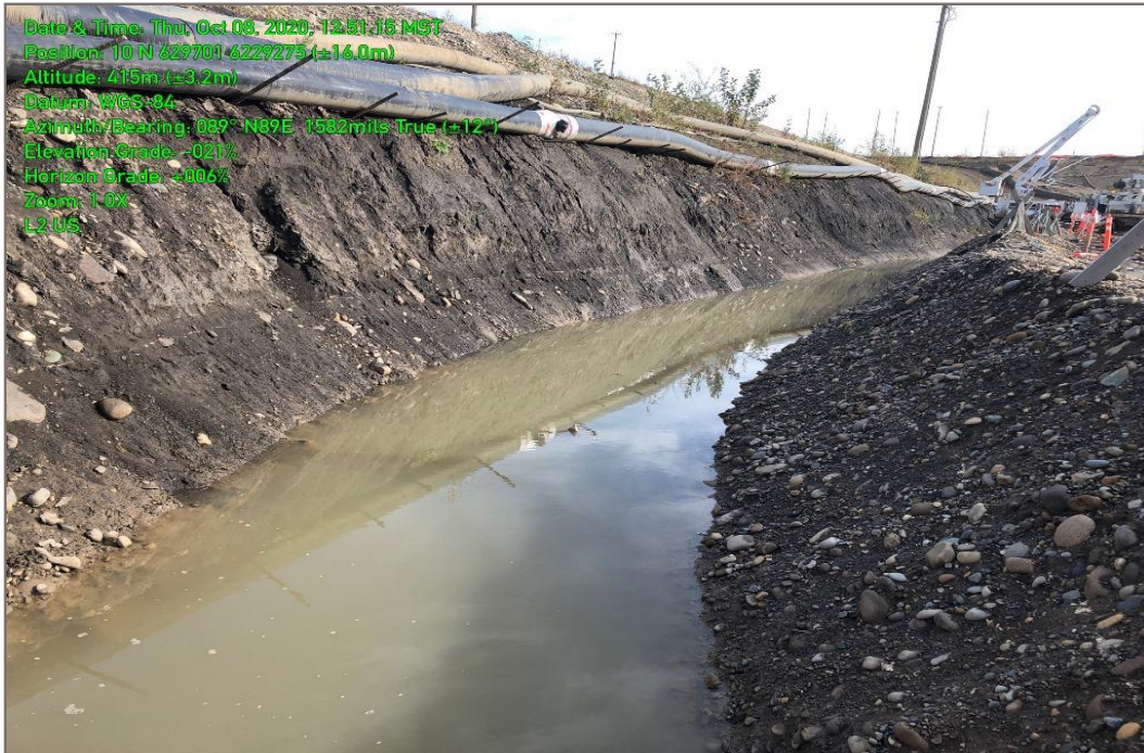
Photo 25: Right Bank L2 Powerhouse Area L2 US upstream location, October 8, 2020.
