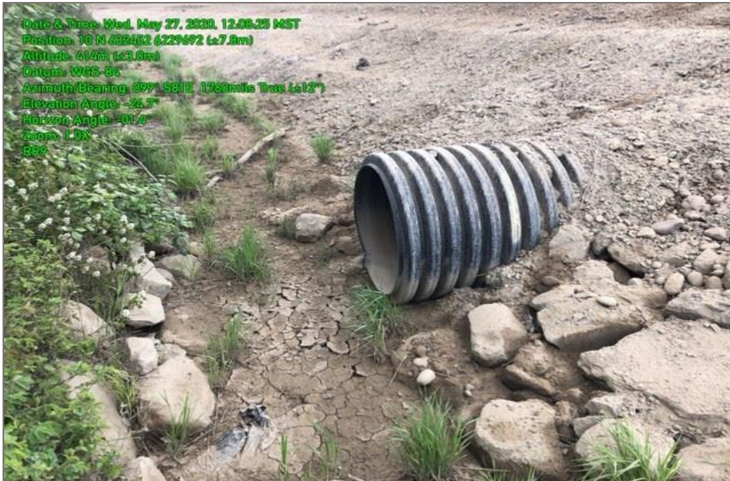
Photo 11: River Road RR9 location, May 27, 2020.
