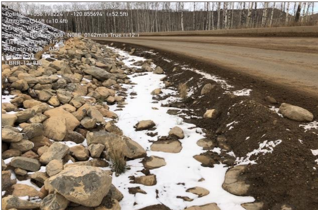
Photo 8: River Road LBRR-12+810 location, October 20, 2020.
