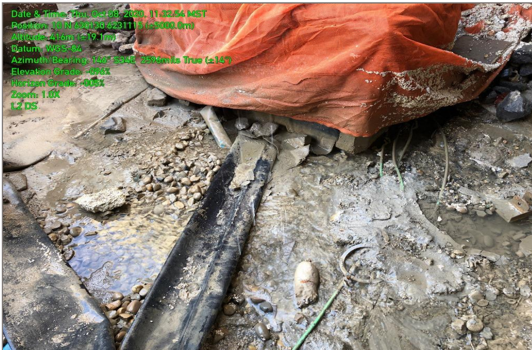
Photo 24: Right Bank L2 Powerhouse Area L2 DS downstream location, October 8, 2020.
