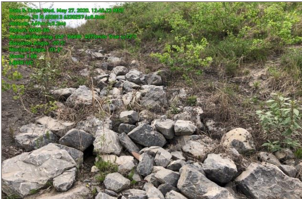
Photo 4: River Road LBRR-UC location, May 27, 2020.
