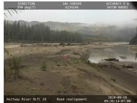
HIGH-CHAIN FROM 19.2-G LOOKING TOWARDS 19.2-F FOR ROAD REALIGNMENT
