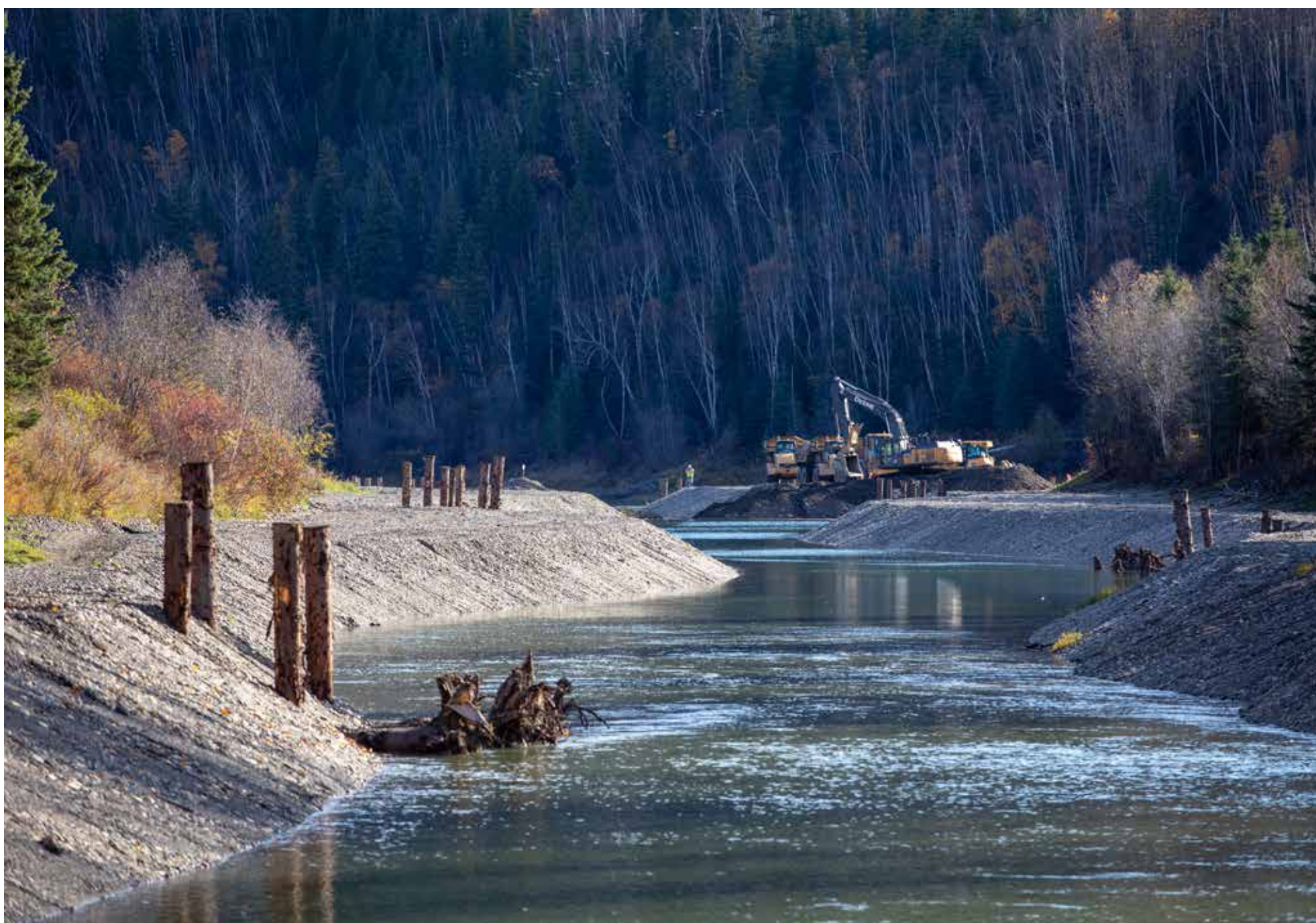
Construction of new downstream channels for fish habitat
