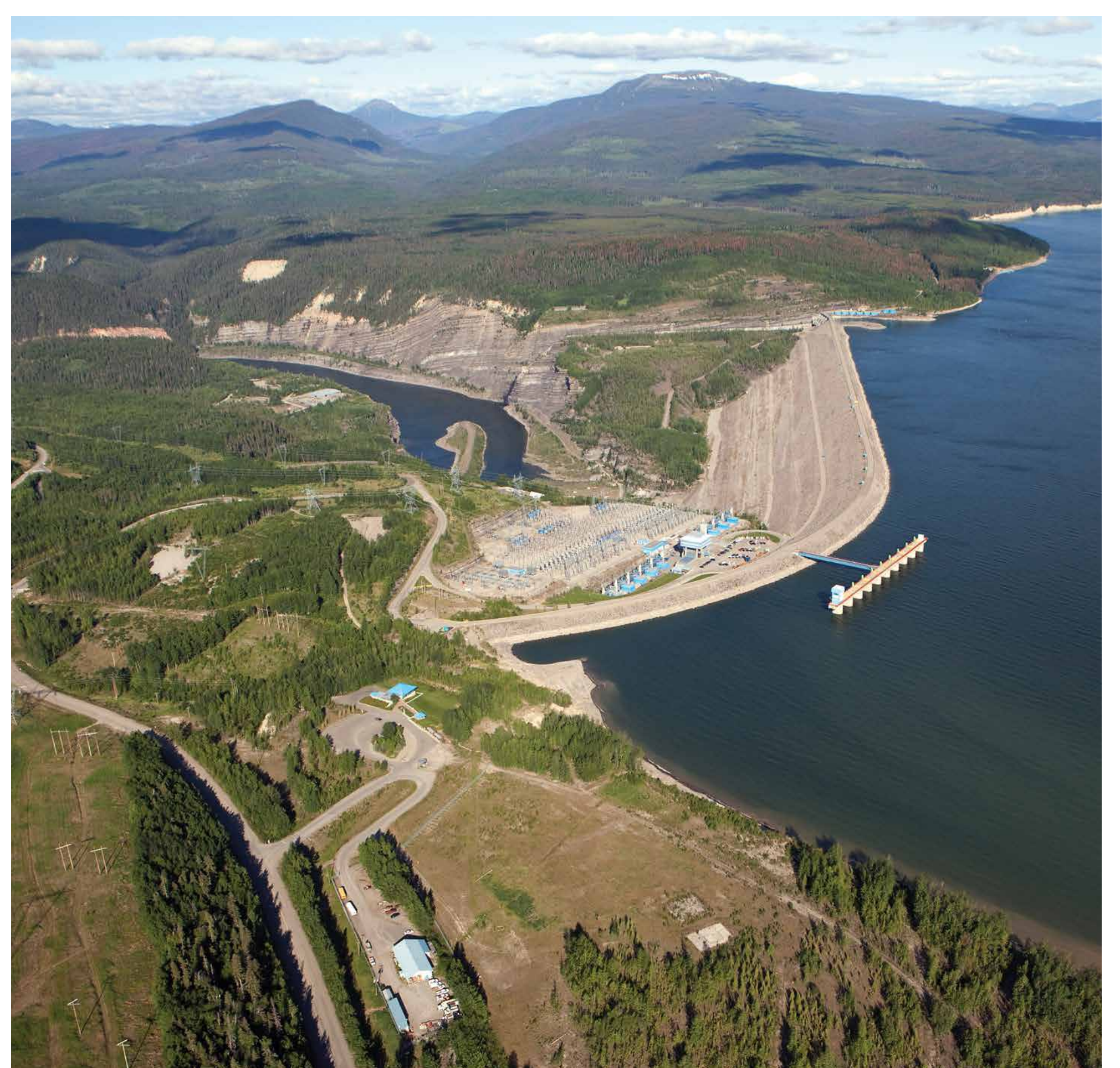
W.A.C. Bennett Dam
