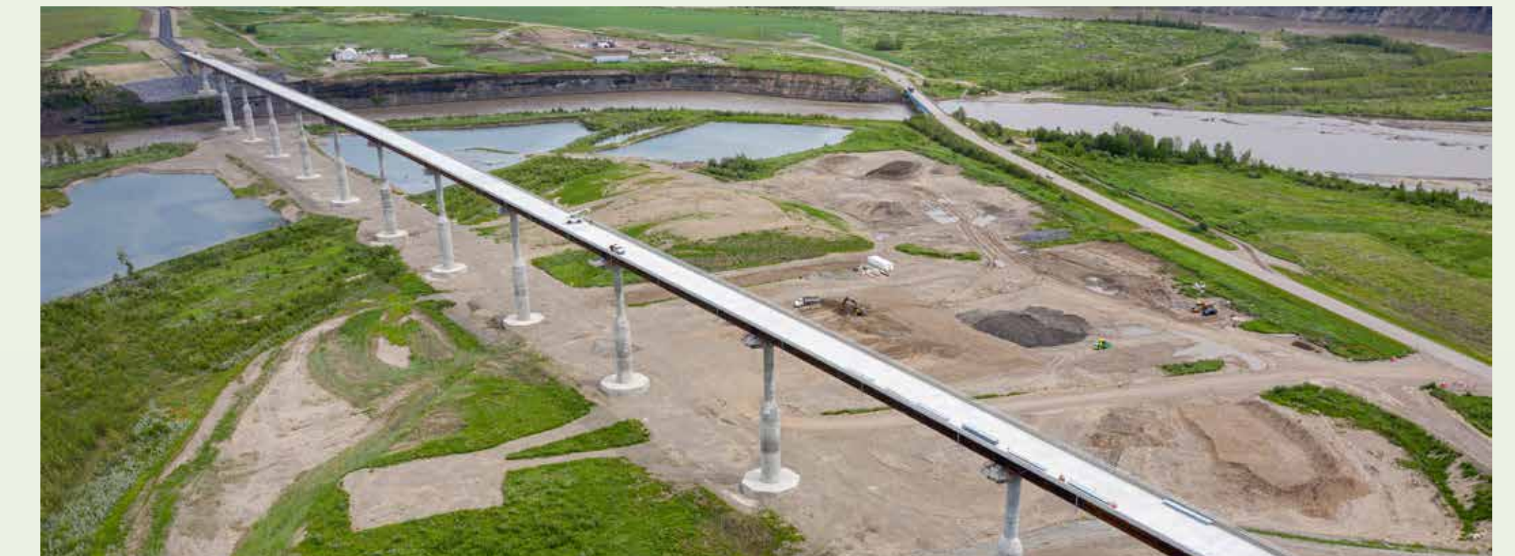
Halfway River bridge
