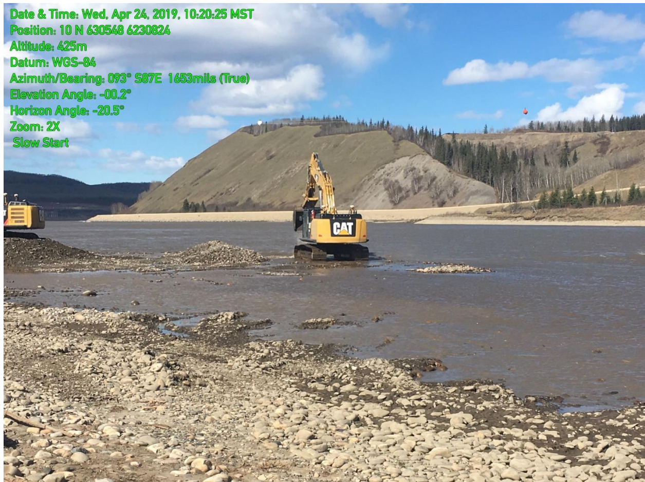
Figure 4. An excavator works to contour a bar in the Peace River at Site 108R to reduce potential for fish stranding. The excavator works in a slow, controlled and continuous manner to scare and exclude fish from the work area (April 24, 2019).
