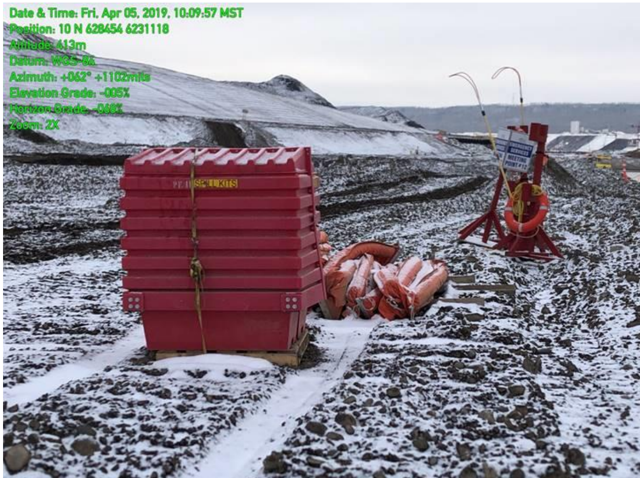
Figure 5. Absorbent and containment booms are on-site and available for deployment in the event of a spill at RSEM L5 (April 5, 2019).
