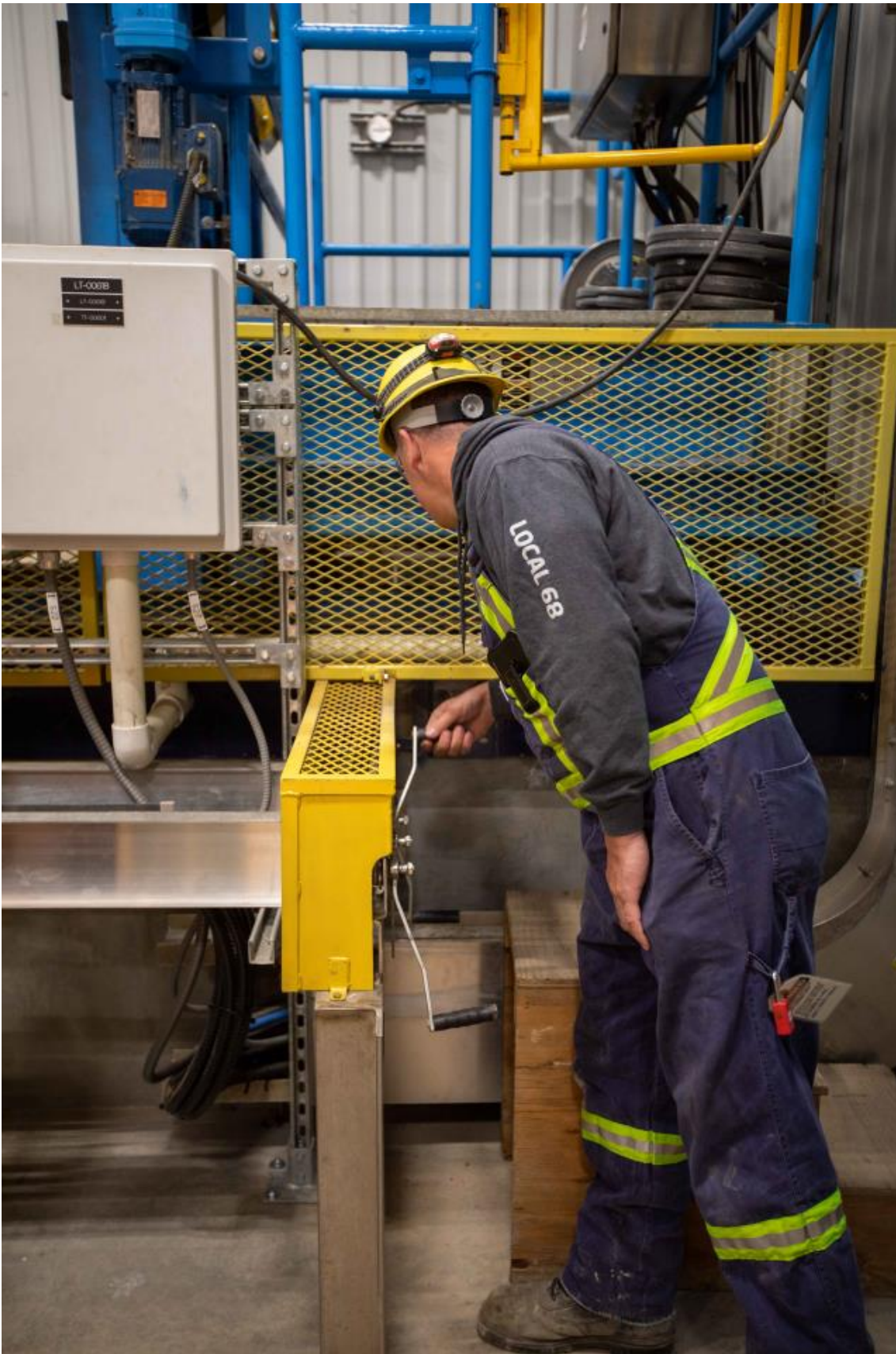
Photo 3. Worker opens the vee-trap on the first day of commissioning (September 23, 2020).
