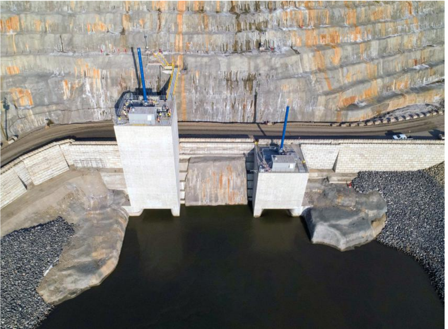
Photo 4. Diversion began on September 30, 2020, when the diversion tunnel gates were opened.
