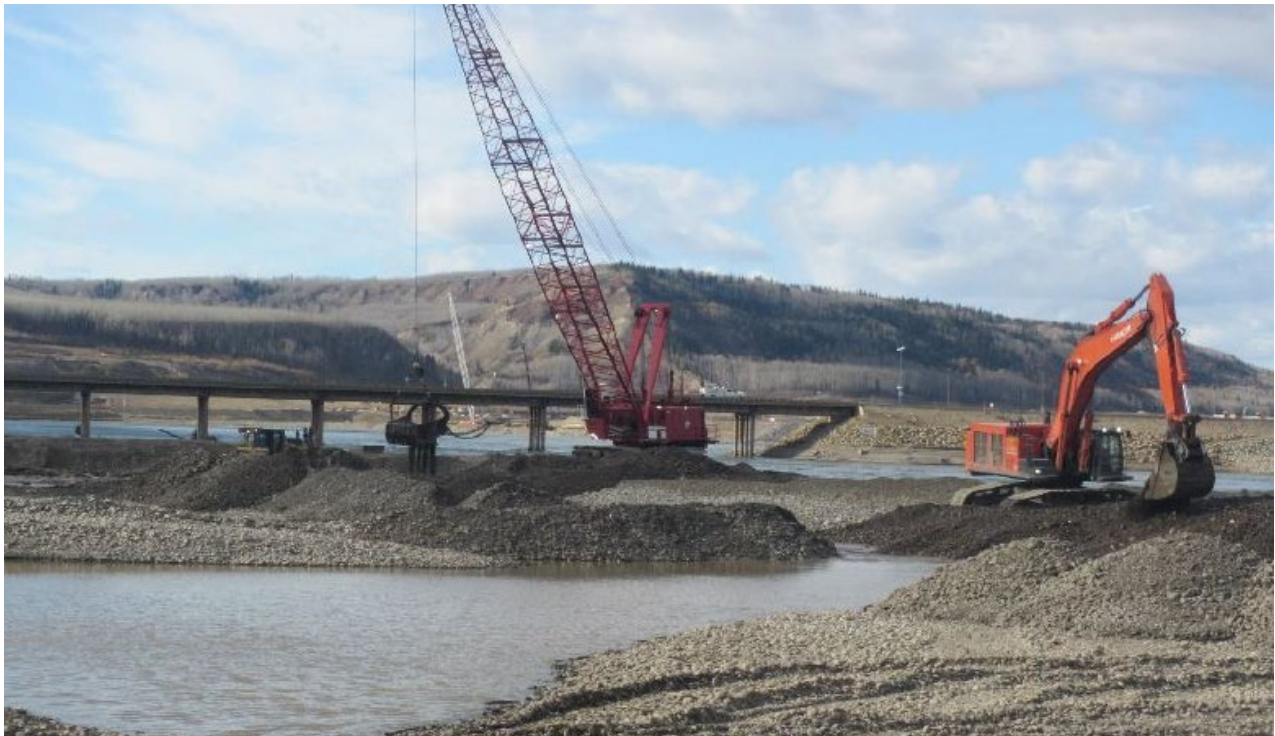
Figure 6. Contouring of Peace River mainstem bar downstream of the dam site (October 5, 2020; from south bank looking west).
