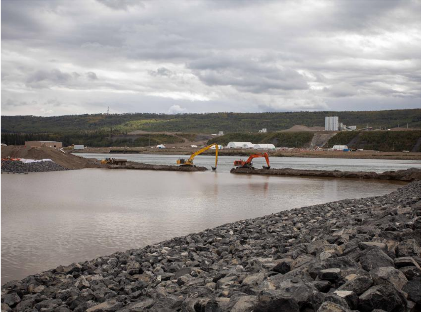
Photo 1. Excavators breach the Stage 1 Downstream Cofferdam to connect the diversion tunnel outlet with the Peace River (September 11, 2020).
