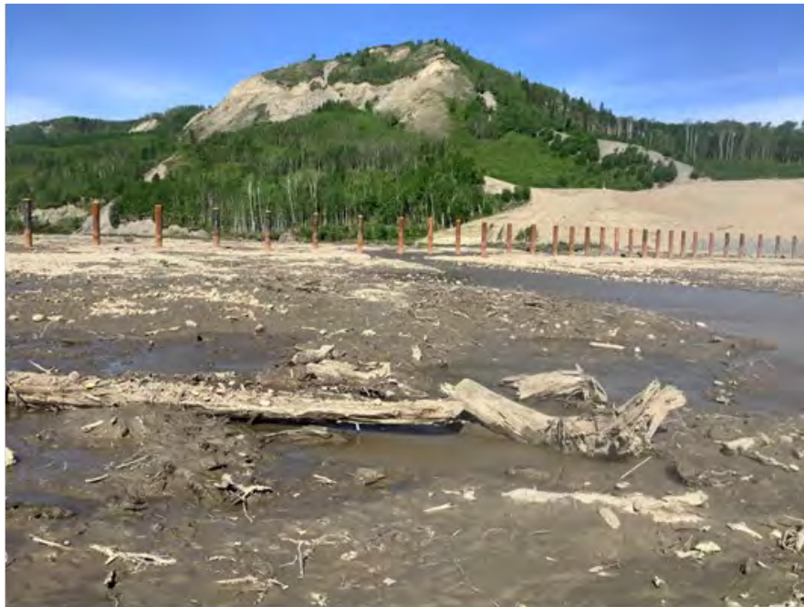
Figure 3. Looking Upstream Moberly right side of channel at MBR-DHSD-SC104.7 on June 1, 2021.
