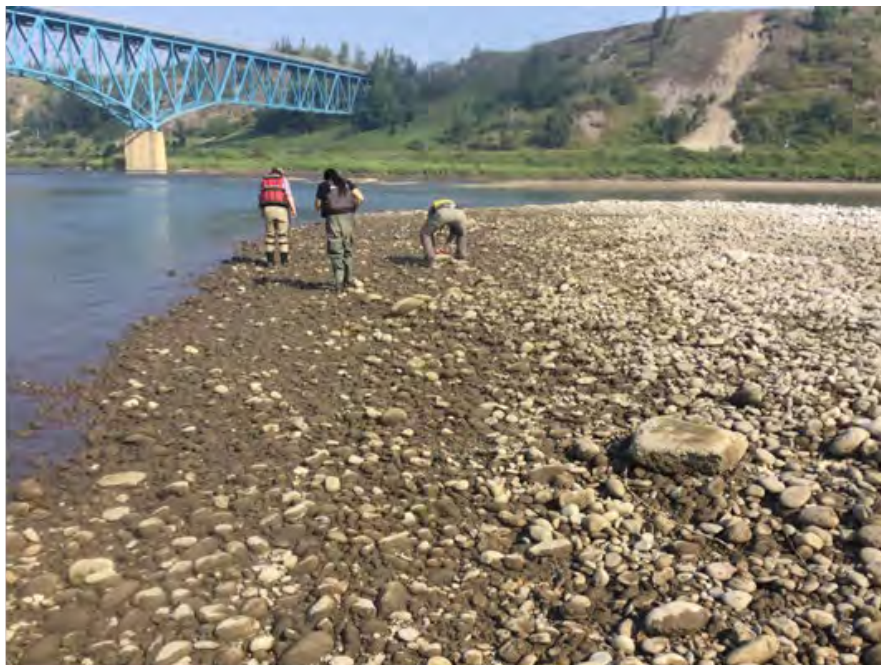
Figure 28. Looking Upstream PCR-R2SD-MC123.5 on August 3, 2021.
