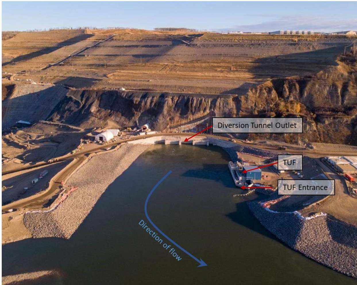
Figure 1.1 Aerial photo of the diverted Peace River and the temporary upstream fish passage facility (TUF) at the Site C Clean Energy Project. The Peace River is diverted through tunnels, which do not provide upstream fish passage. Photo provided by BC Hydro, June 8, 2021.
