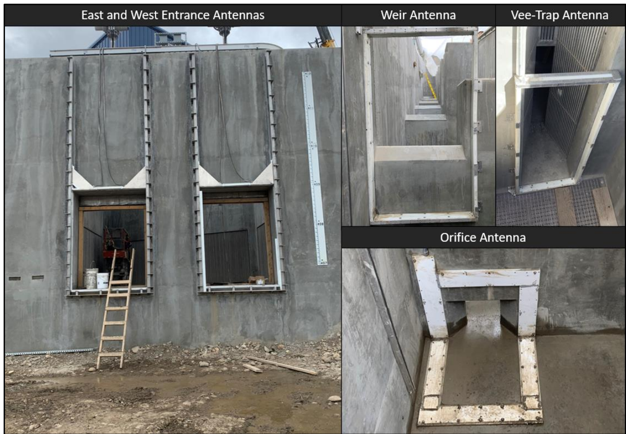
Figure 2.4 Photos of completed PIT antennas installed within the dewatered temporary upstream fish passage facility prior to operations.
