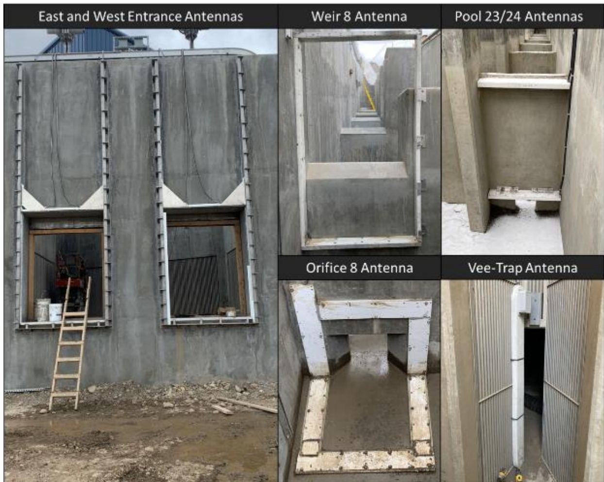
Figure 7. Photos of completed PIT antennas installed within the dewatered temporary upstream fish passage facility prior to operations.
