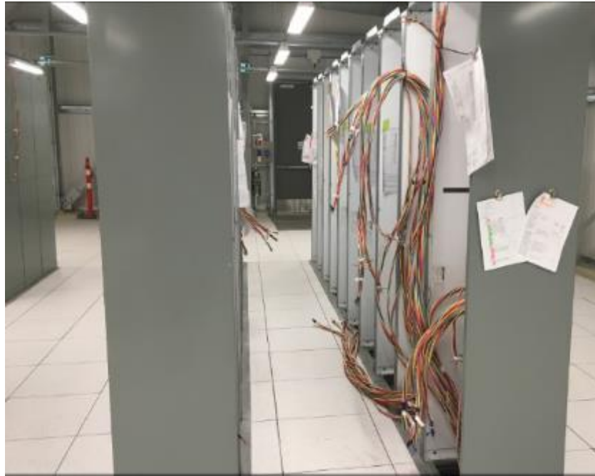
Control Building – Cable Stripping
