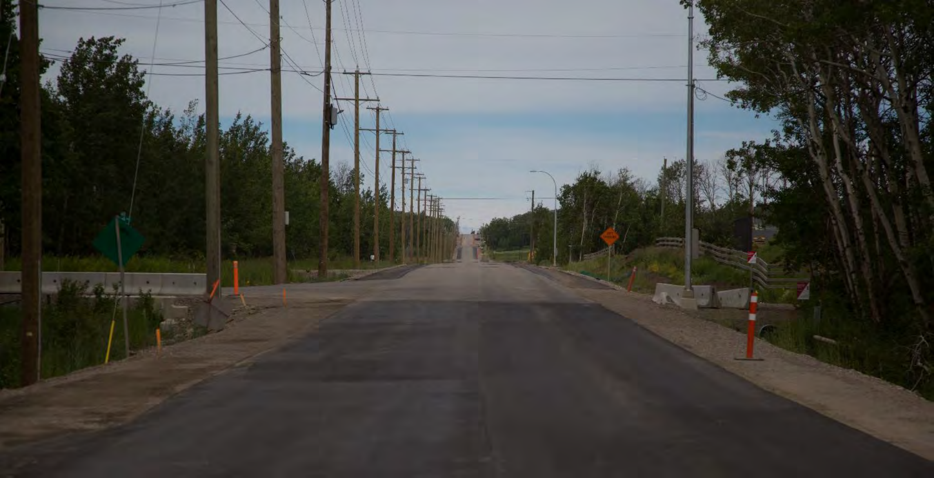
Old Fort Road Repaving and Shoulder Widening
