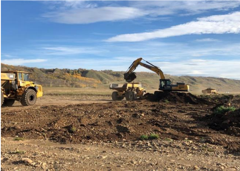
Halfway River site preparation September 21, 2019
