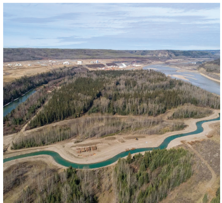
Newly-built channels provide fish habitat enhancements
