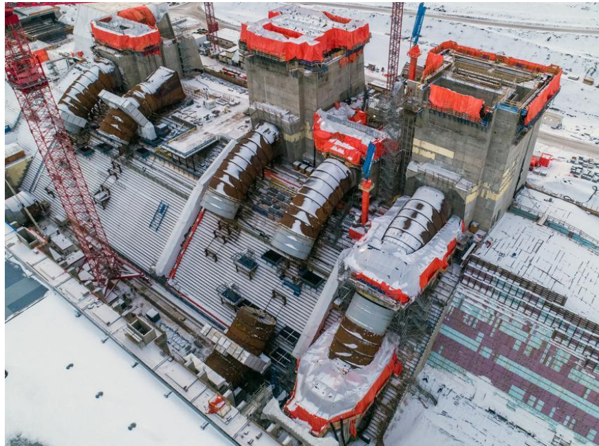
Figure A-1 An aerial view of the Site C penstocks and intakes under construction (January 2021)
