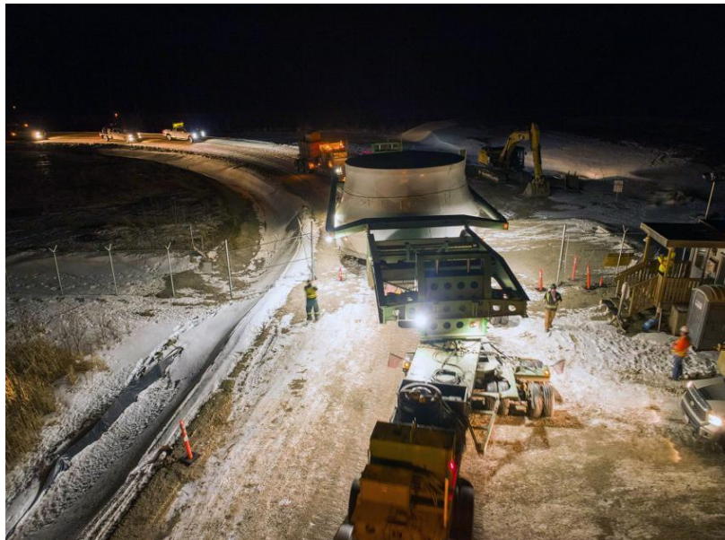
Figure A-2 Unit 1 turbine runner arrives at Site C after travelling from Sao Paulo, Brazil, by ship to Prince Rupert, and transported on a customized truck to the project site (January 2021)
