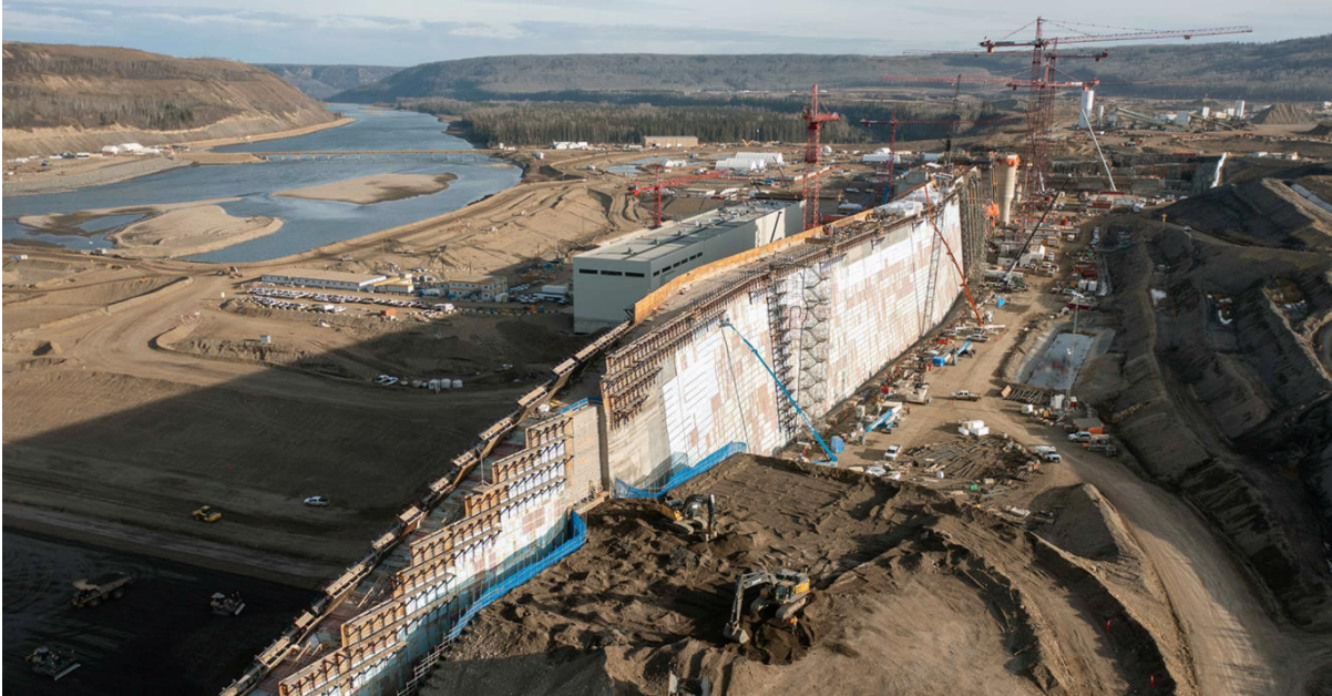
Figure A-21 Roller-compacted concrete buttress (October 2021)
