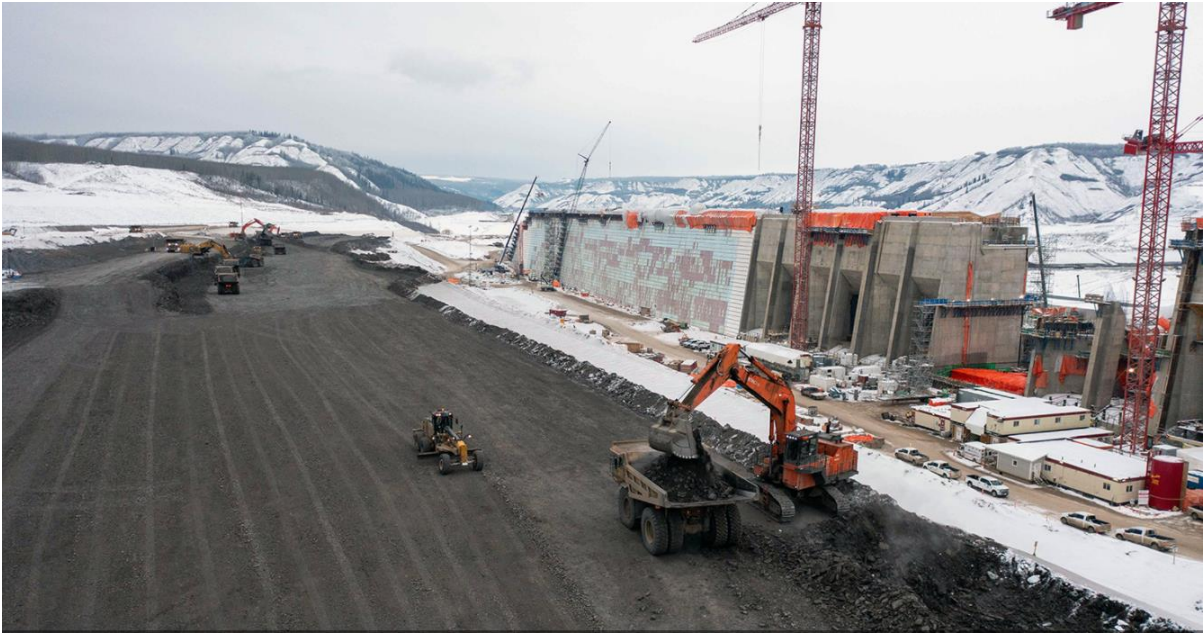
Figure A-26 Approach channel (December 2021)
