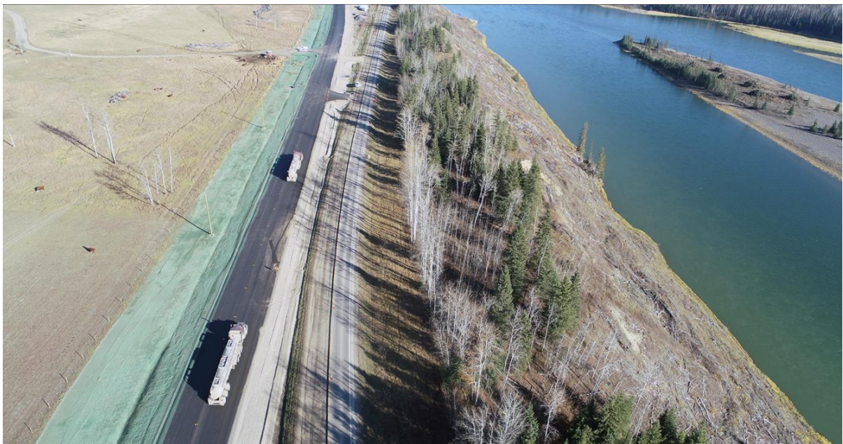
Figure A-20 Highway 29 at Farrell Creek East (October 2021)
