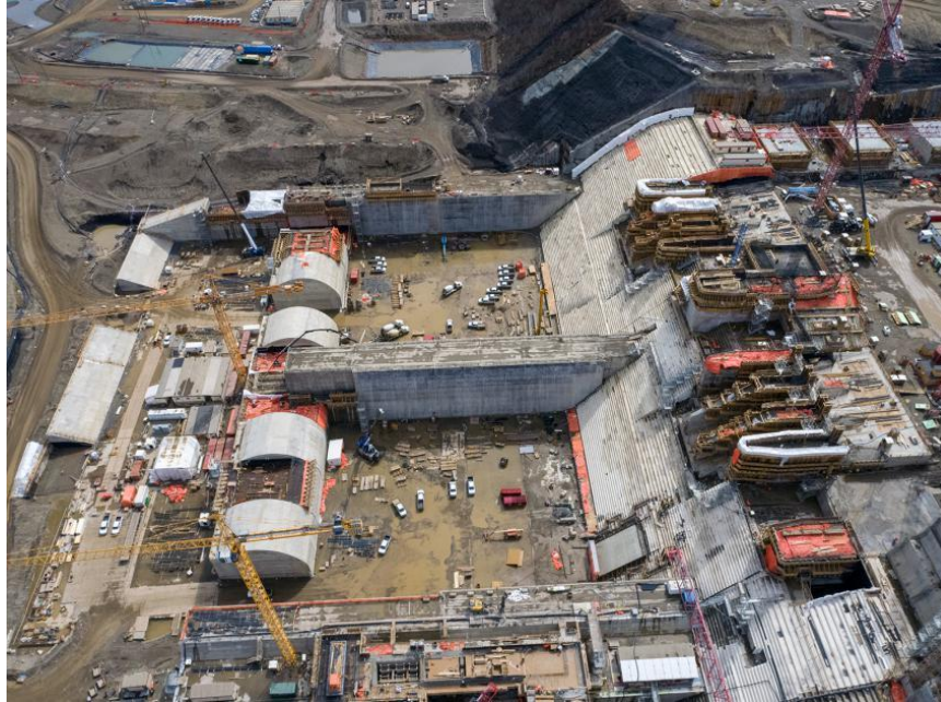
Figure A-7 The spillways, headworks and stilling basins (April 2021)
