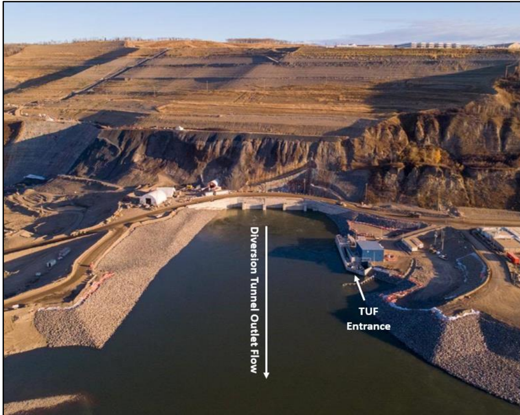
Figure 1 Aerial photo of the diverted Peace River and the temporary upstream fish passage facility (TUF) at the Site C Clean Energy Project, located on the east bank of the diversion tunnel outlet. The Peace River is diverted through two tunnels which do not allow for upstream fish passage. Photo provided by BC Hydro, June 8, 2021.
