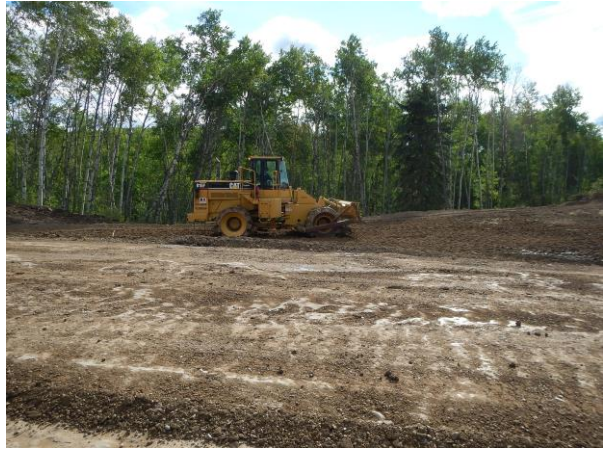
Figure 4: Early road construction – levelling and grading
