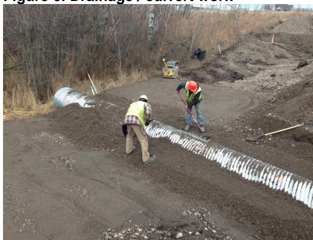
Figure 6: Drainage / culvert work
