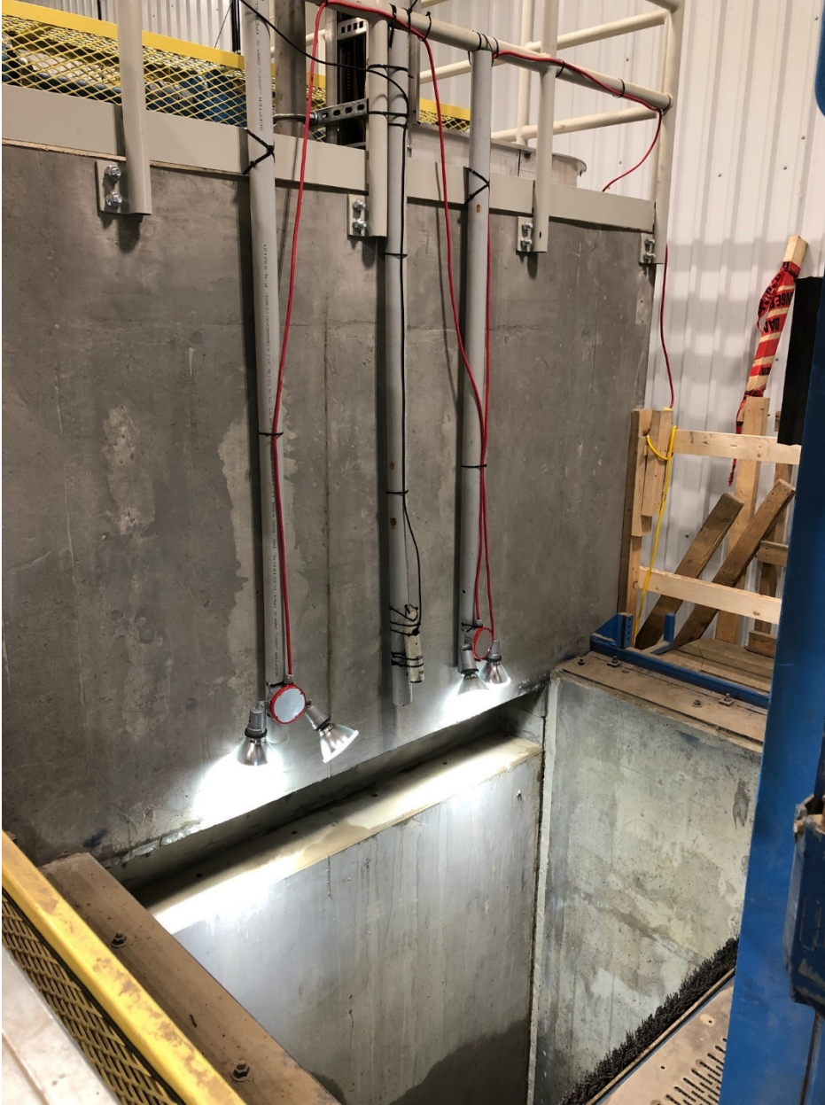
Photo 4. Overhead light and camera system at the upstream end of the pre-sort holding pool (August 16, 2021).
