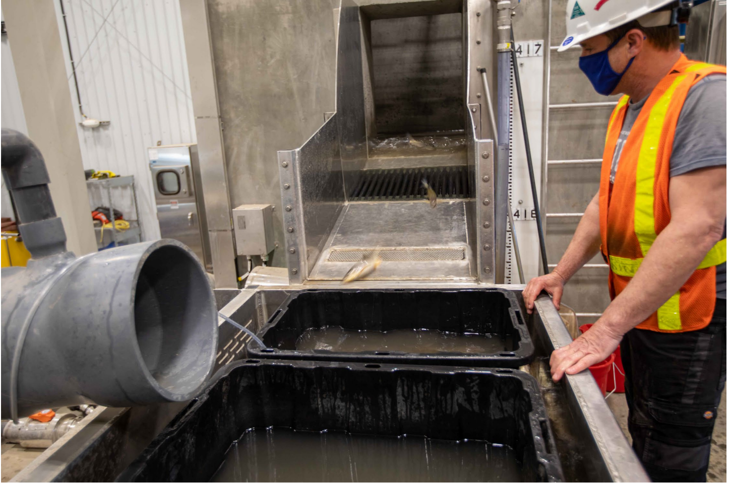
Photo 2. Fish exit a lock into an anaesthetic tank prior to sampling and tagging in the sorting facility (June 21, 2021).
