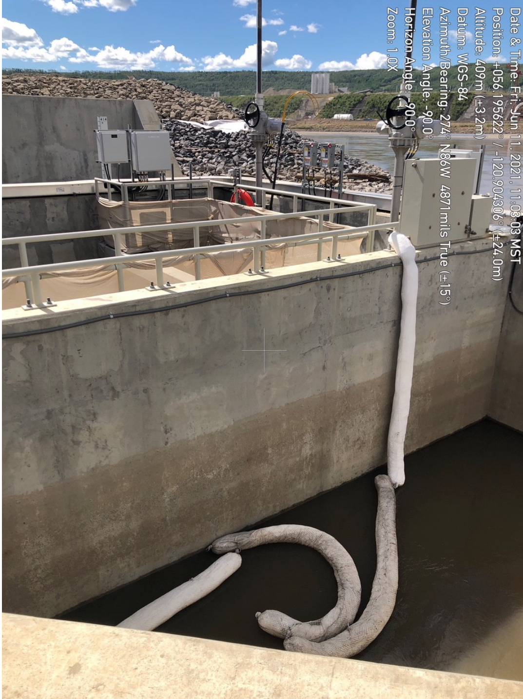
Photo 4. An absorbent boom was deployed in the West AWS Receiving Pool and the entrance gates were closed to mitigate the risk of oil being released into the Peace River (June 11, 2021). Laboratory analysis of the water sample confirmed that the sheen was not hydrocarbon-based and was instead of natural origin.
