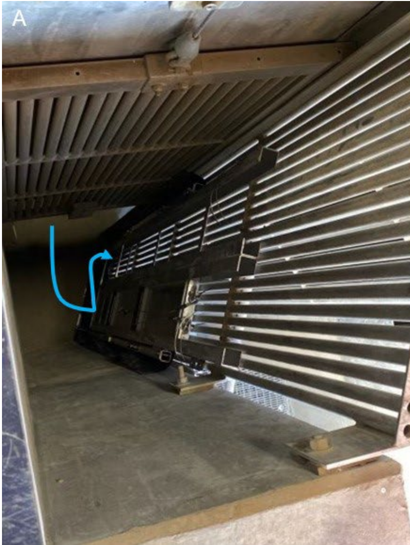
Photo 1. (A) Channels were bolted onto the side arms of the vee-trap and panels were lowered into place to concentrate the flow cue (light blue arrow) through the upstream half of the vee-trap (March 18, 2022). (B) Screenshot of IFC Construction Drawing 1020-M13-00419 showing the vee-trap and spatial context of (A).
