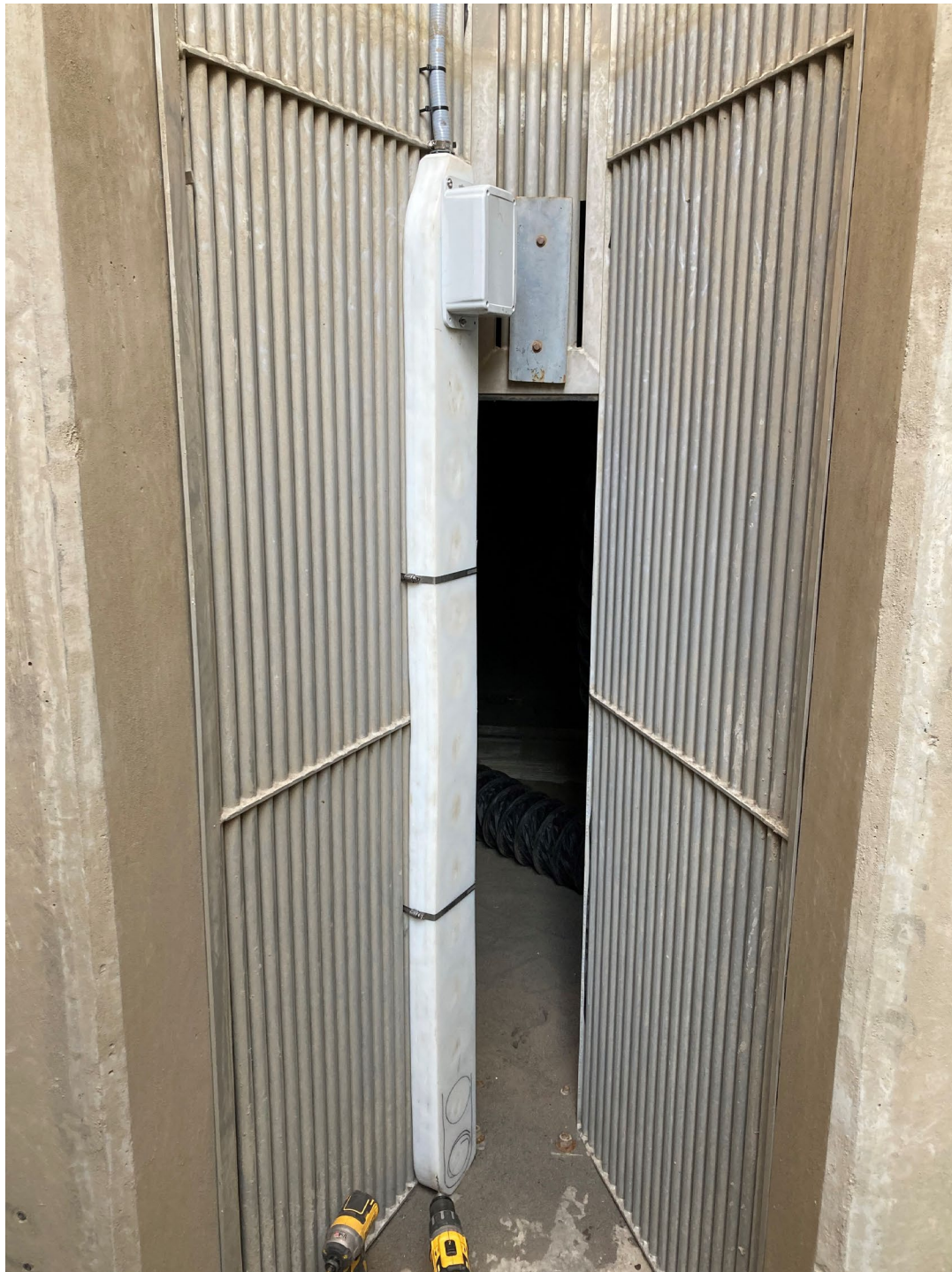
Photo 3. Crews install a passive integrated transponder (PIT) antenna onto the side of the vee-trap to detect tagged fish entering the pre-sort holding pool (March 18, 2022).
