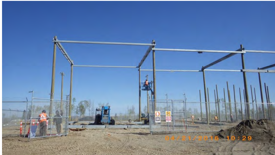
Figure A-19 Temporary Substation being Erected (April 2016)
