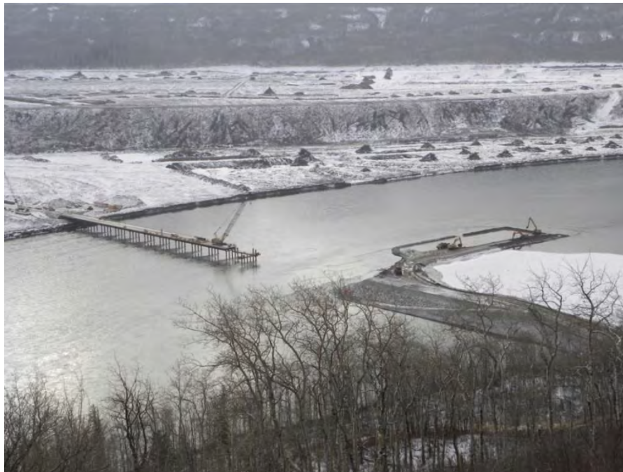
Figure A-9 Temporary Construction Access Bridge Partially Built (February 2016)
