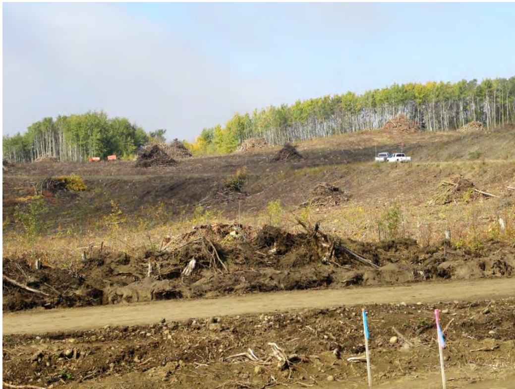
Figure A-2 Clearing in Progress at Dam Site (August 2015)
