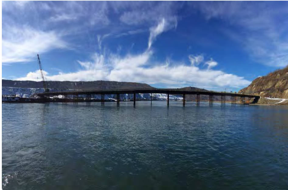
Figure A-10 Peace River Construction Bridge in Service (April 2016). The Bridge was Completed on Time and on Budget by Ruskin Construction and a First Nations Joint Venture Partner
