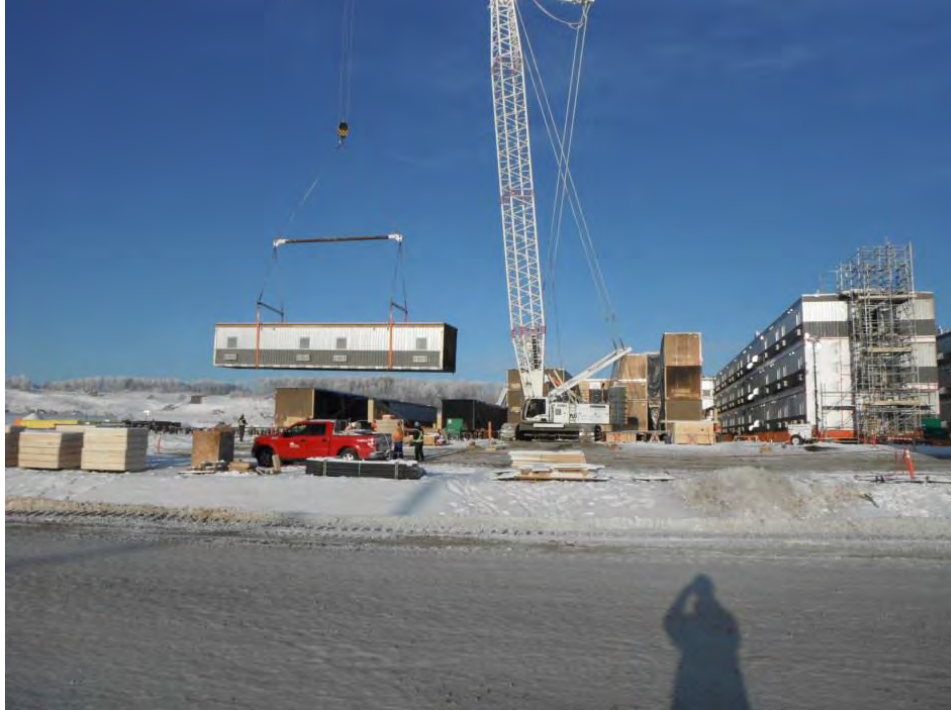
Figure A-11 Worker Accommodation Lodge under Construction (December 2015)
