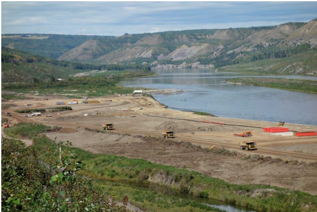
Figure A-27 Right Bank Cofferdam Preparation (August 2016)
