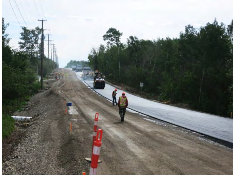
Figure A-16 Upgrading Continues on 240 Road (June 2016)
