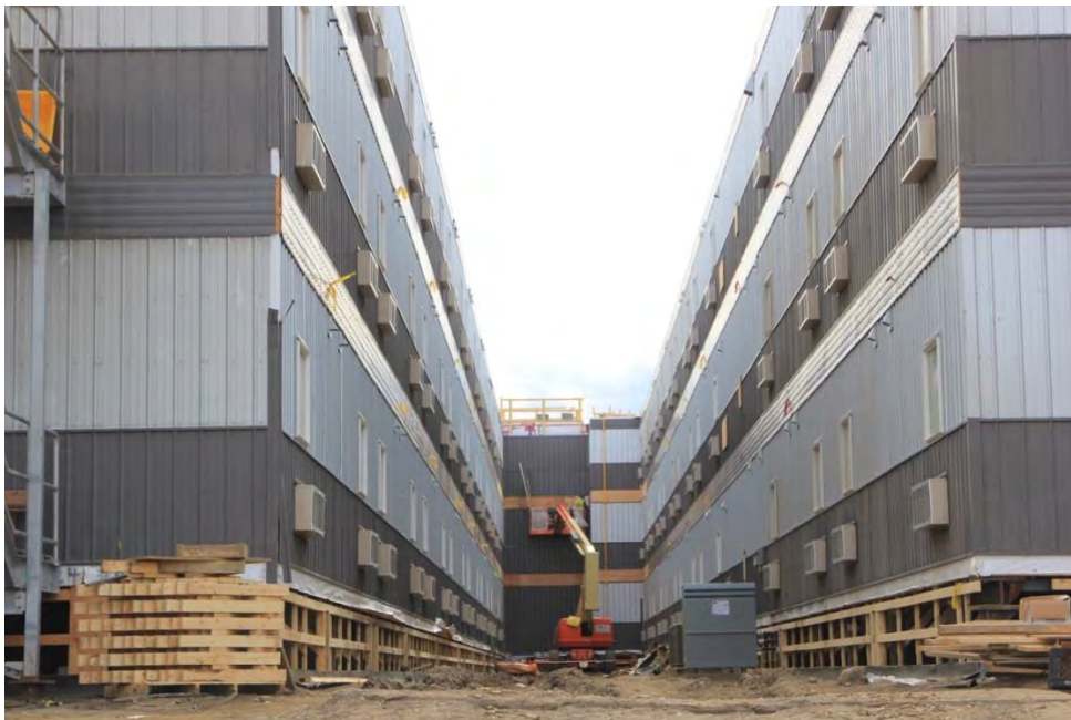
Figure A-12 Work Continues on the Worker Accommodation Lodge (April 2016)
