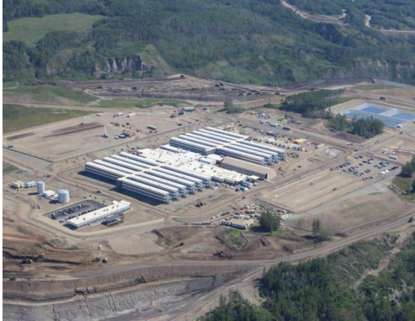
Figure A-8 Aerial View of North Bank of Dam Site Showing the Worker Accommodation Lodge (July 2016)
