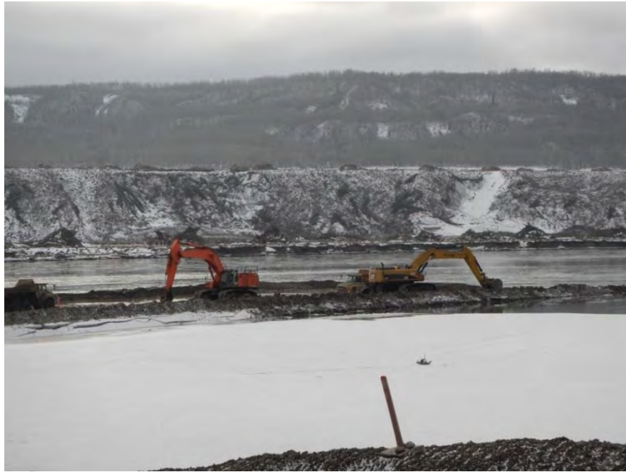
Figure A-12 In River Excavation (February 2016)
