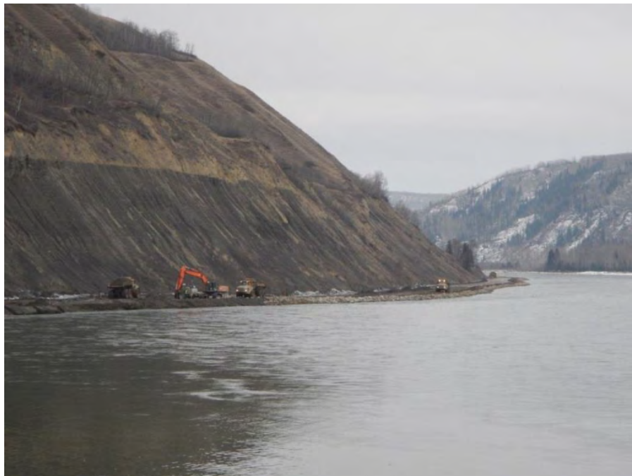
Figure A-13 Placing Rip-Rap on River Road (May 2016)
