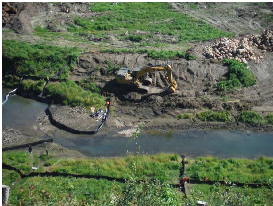
Figure A-23 Excavator Preparing Area at Right Bank Drainage Tunnel (July 2016)
