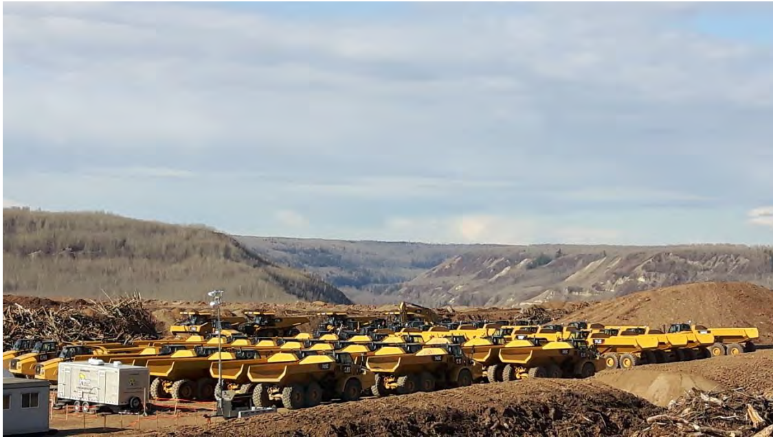
Figure A-21 Peace River Hydro Partners Preparing to Mobilize to Site (April 2016)
