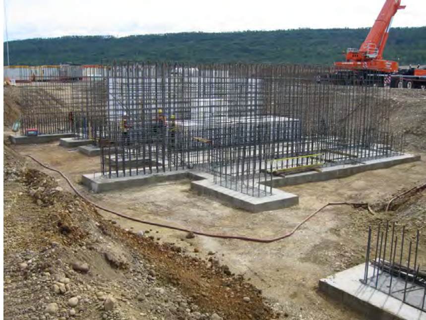
Figure A-24 South Foundation for Roller-Compacted Concrete Batch Plant (July 2016)
