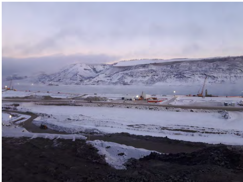
Figure A-9 Excavation Continues for the South Bank Approach Channel (January 2017)
