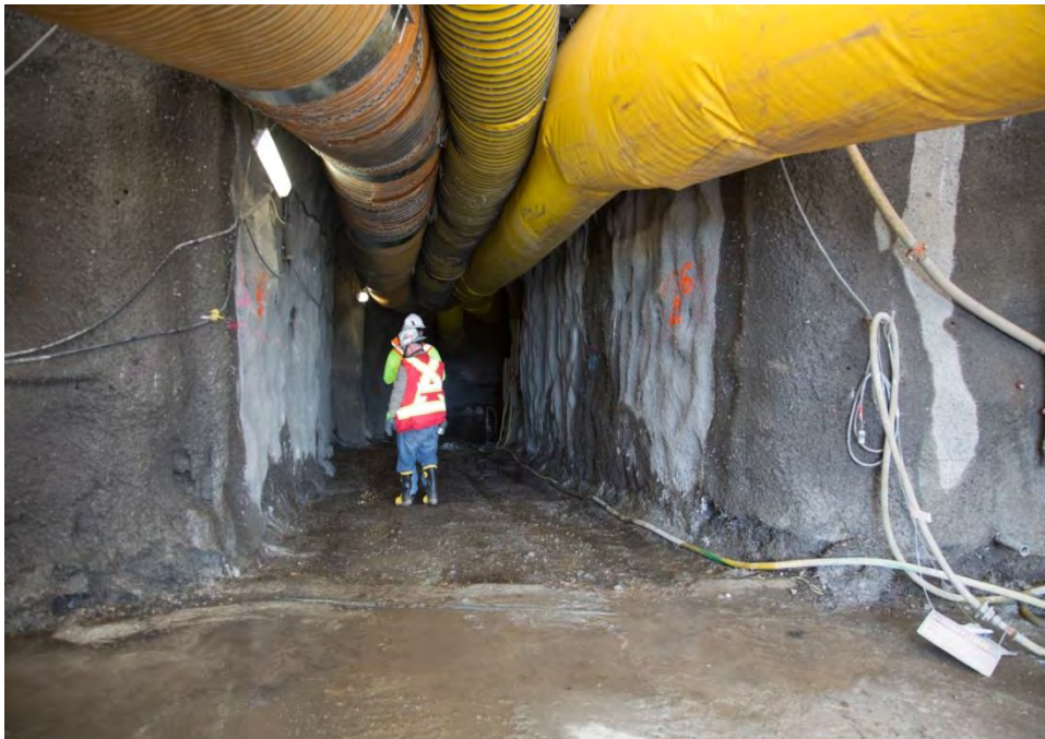
Figure A-16 South Bank Drainage Tunnel (May 2017)
