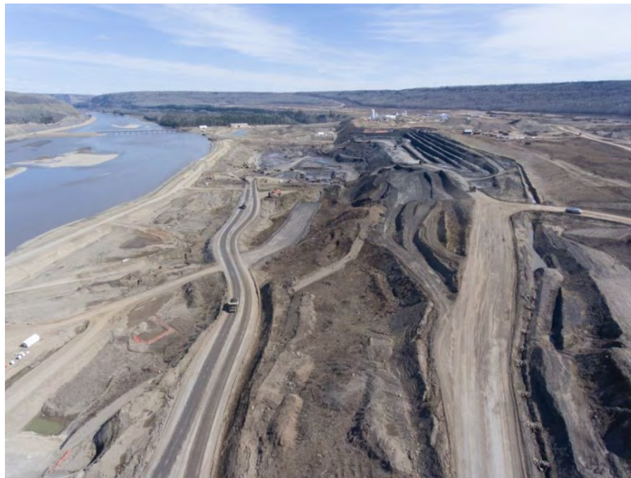
Figure A-14 South Bank Approach Channel and Buttress Excavation (May 2017)
