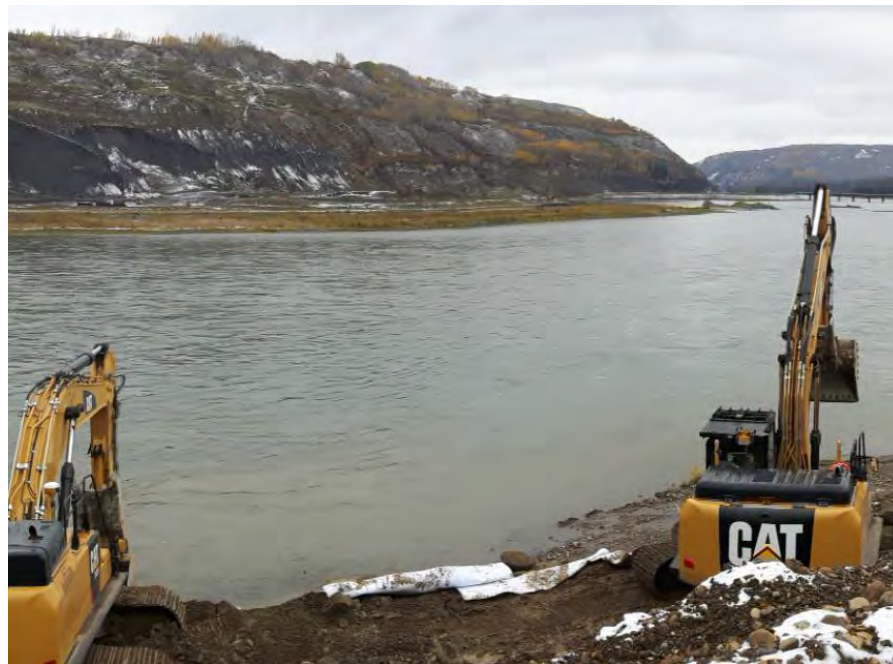
Figure A-12 Riprap Placement along the South Bank Cofferdam (April 2017)
