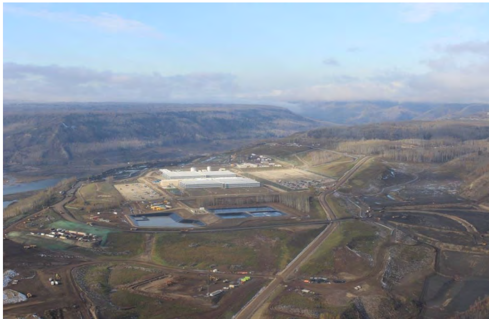
Figure A-4 Completed Worker Accommodation Lodge, Looking West. (October 2016)
