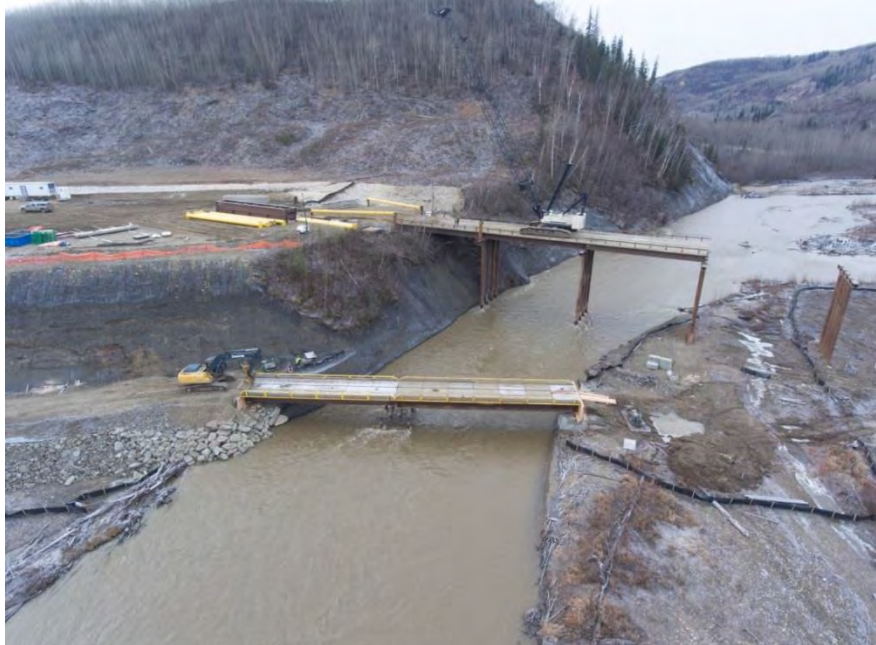
Figure A-6 Construction Continues on the Moberly River Construction Bridge (November 2016)
