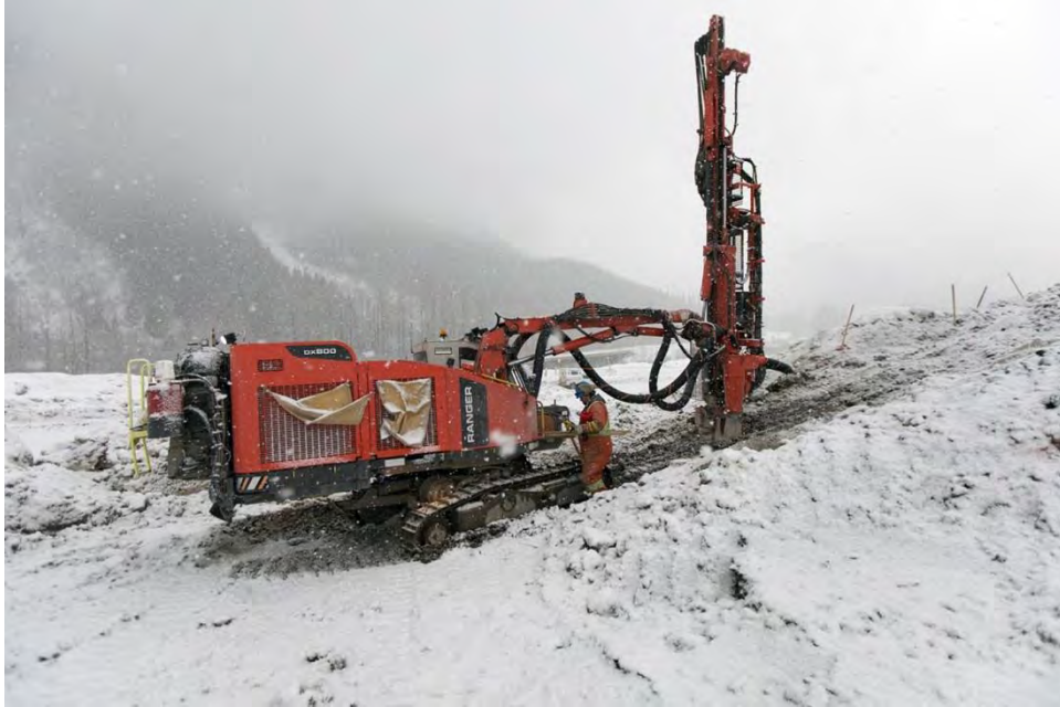
Figure A-34 Drilling at West Pine Quarry (November 2017)
