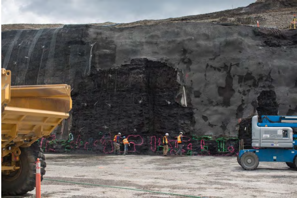
Figure A-19 Rock Slope Stabilization at the Stilling Basin (June 2017)
