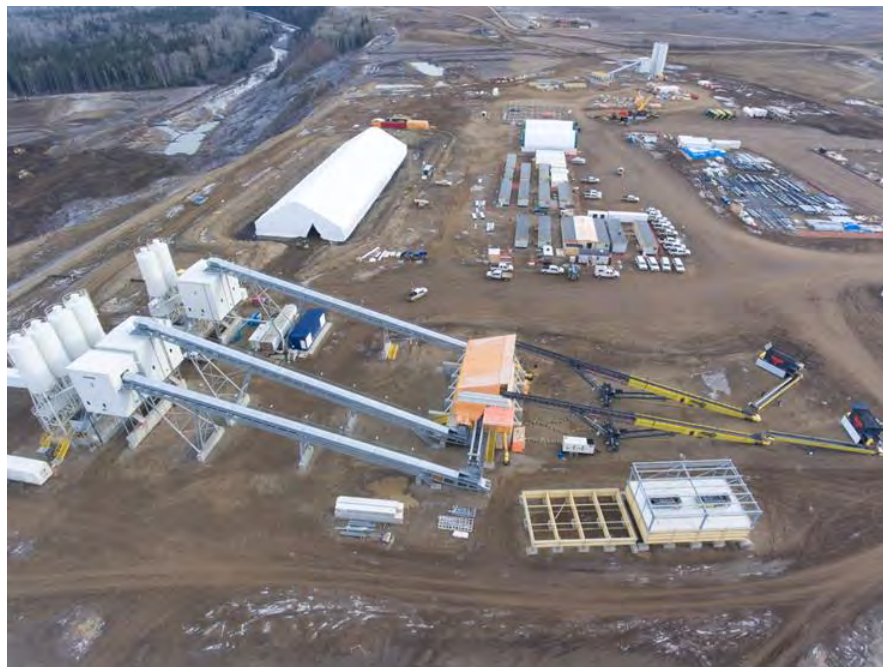
Figure A-7 Concrete Batch Plant on the South Bank (November 2017)
