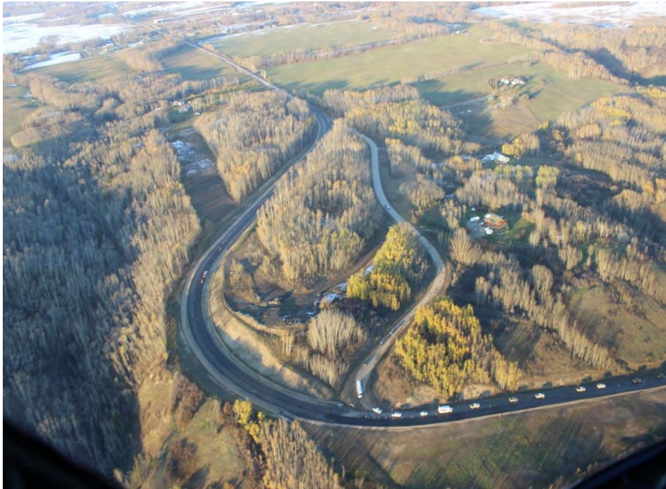
Figure A-3 Old Fort Road Realignment (October 2016)
