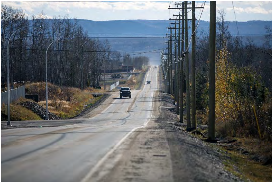
Figure A-28 Completed Upgrades to Old Fort Road (October 2017)
