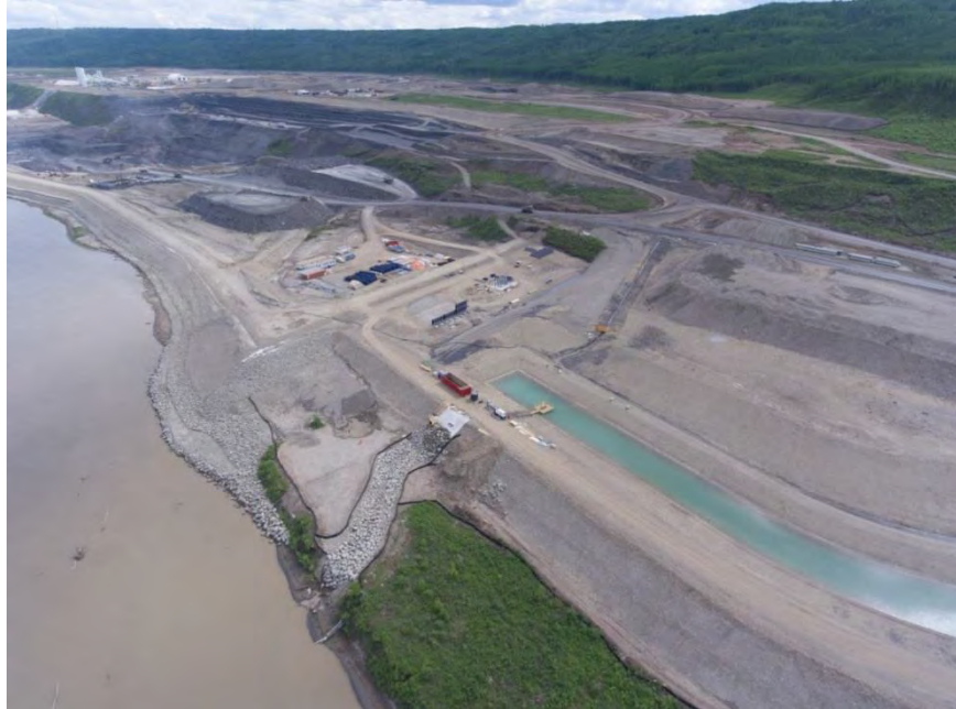
Figure A-17 South Bank Cofferdam, Excavation, and Sediment Storage Area. (May 2017)
