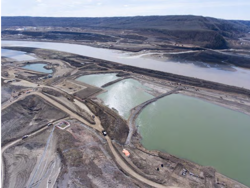
Figure A-15 North Bank Excavation, Looking South East (May 2017)
