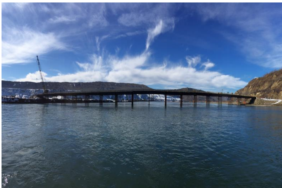
Figure A4 Peace River Construction Bridge in Service
