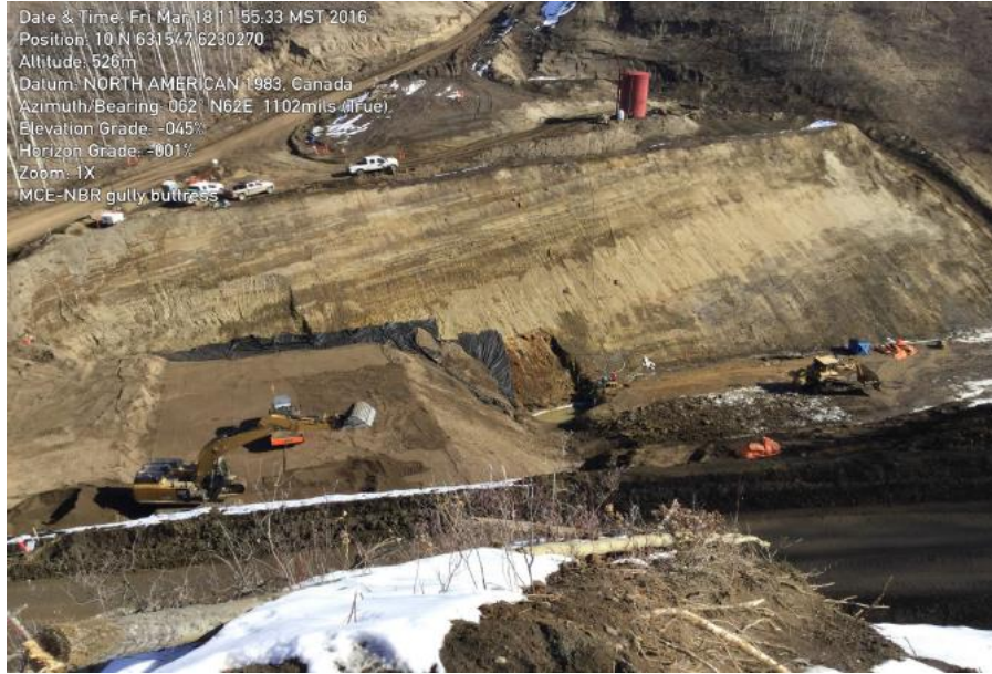
Figure A-1 Construction of the L3 Gully Buttress
