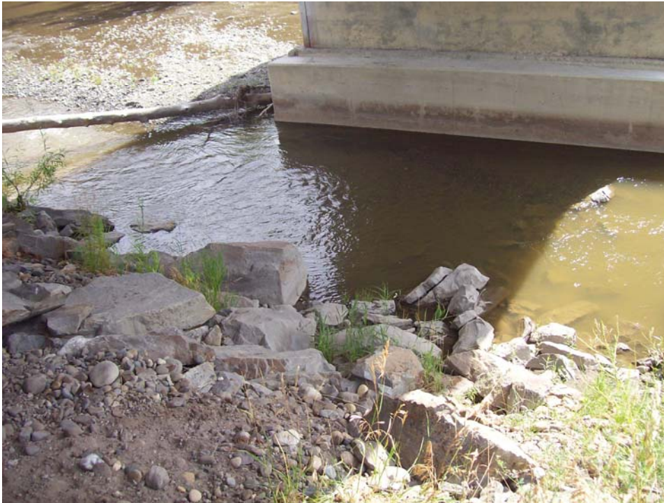
Photo 32. Rip rap bank of Farrell Creek at Highway 29 Bridge.
