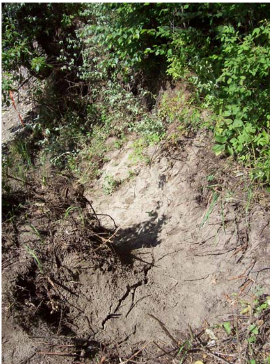
Photo 95. Secondary bank trail from Rat Camp to shoreline (dug out stairs).
