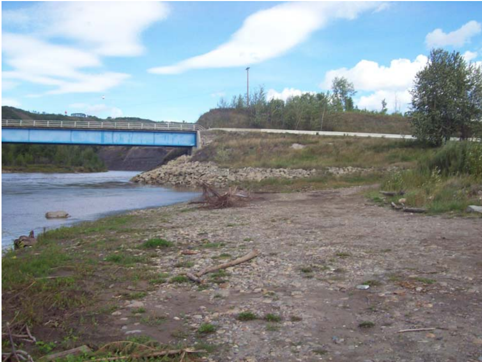
Photo 37. Halfway River Bridge boat launch.
