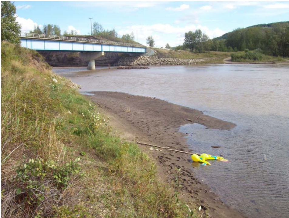
Photo 39. Shoreline access (of the Halfway River) from west side of the Halfway River Bridge looking east.
