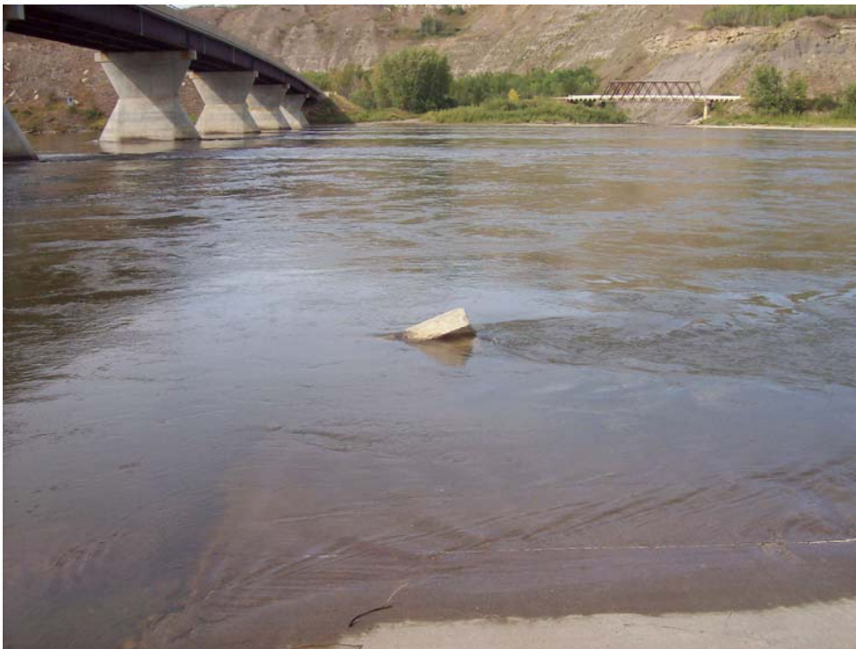
Photo 81. Blackfoot park potential hazard: large piece of concrete at end of boat launch.
