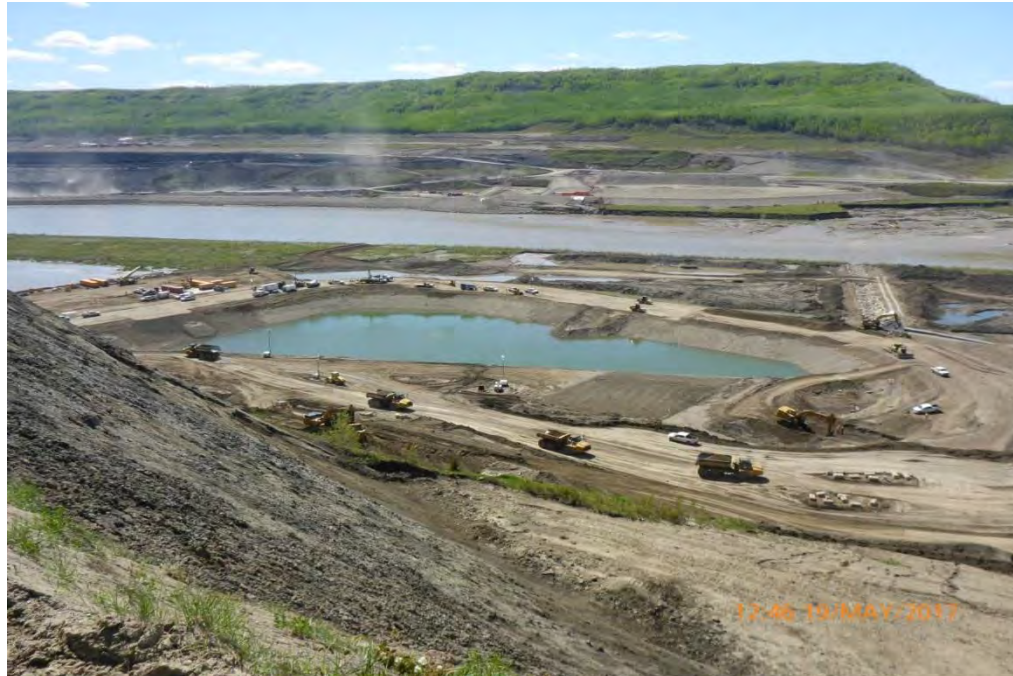
Figure A-5 Inlet Cofferdam Overview. Photo taken May 19, 2017.
