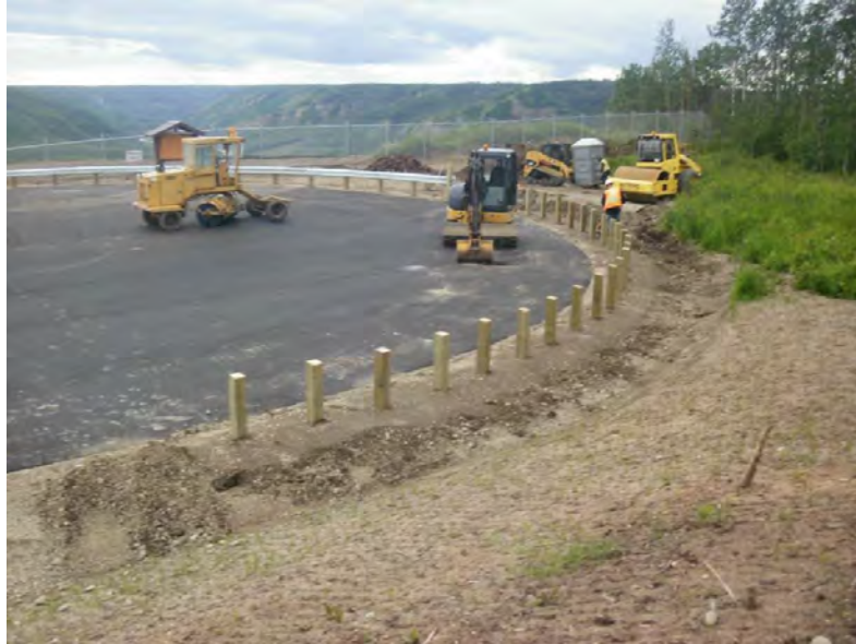
Figure A-11 View Point – Guardrail Installation. Photo taken June 18, 2017.
