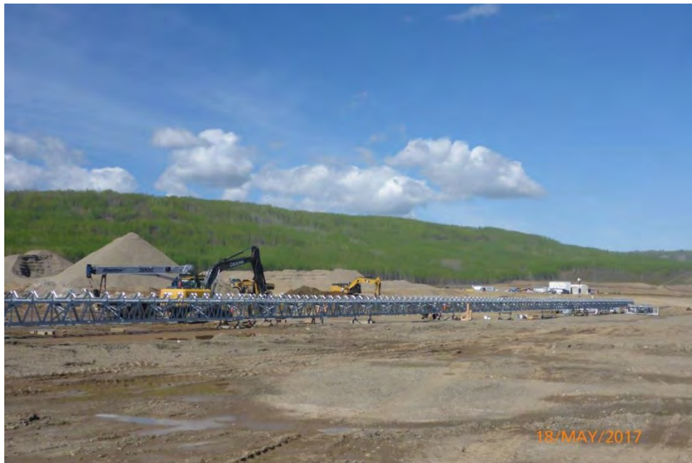
Figure A-4 Area 20 – Roller-Compacted Concrete Conveyor Construction. Photo taken May 18, 2017.
