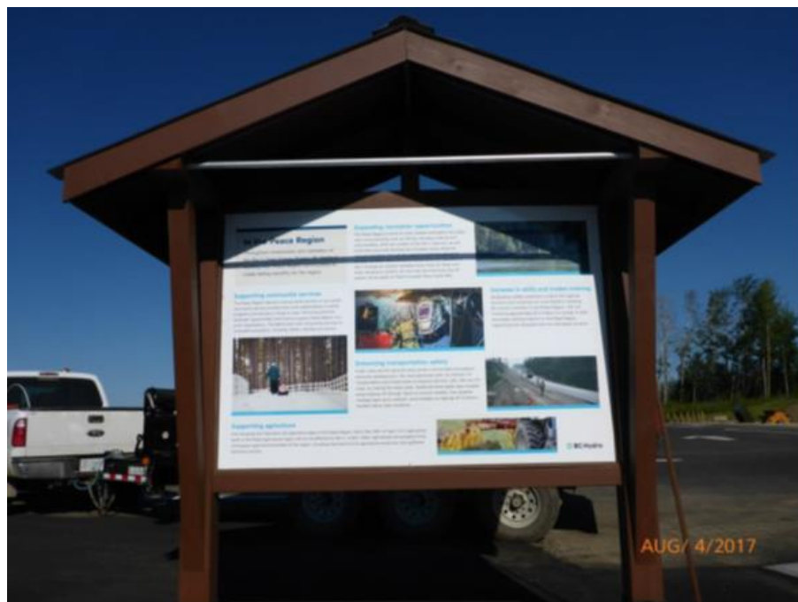
Figure A-6 Installation of Viewpoint Sign No. 4. Photo taken August 4, 2017.
