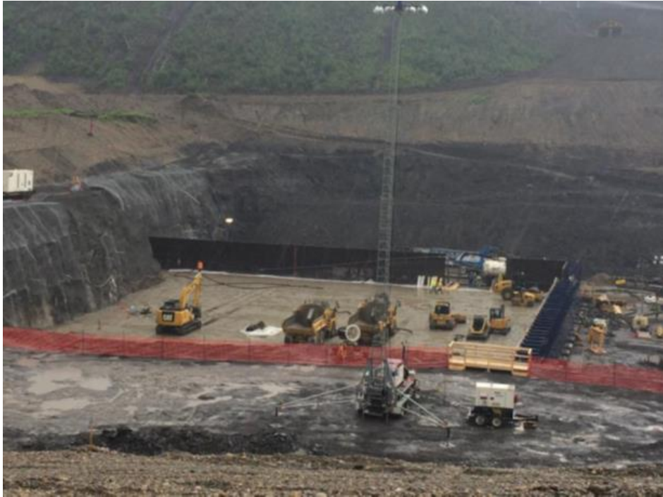
Figure A-1 Right Bank Excavation Stilling Basin. Photo taken July 13, 2017.
