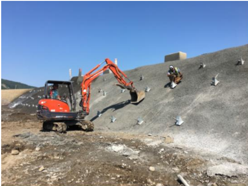
Figure A-2 Right Bank Excavation (Tailrace). Photo taken July 21, 2017.
