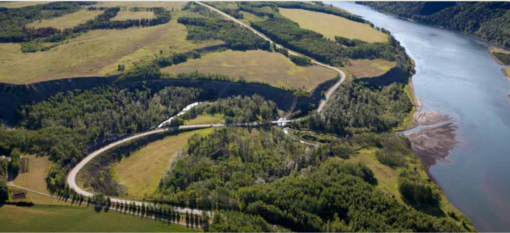
Highway 29 crossing at Farrell Creek
