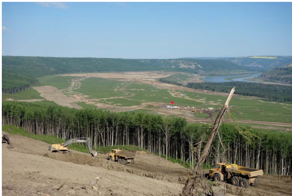
Figure A-6 Right Bank Viewed from Septimus Road
