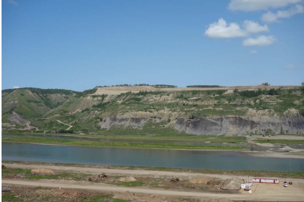
Figure A-3 Left Bank Excavation viewed from Right Bank
