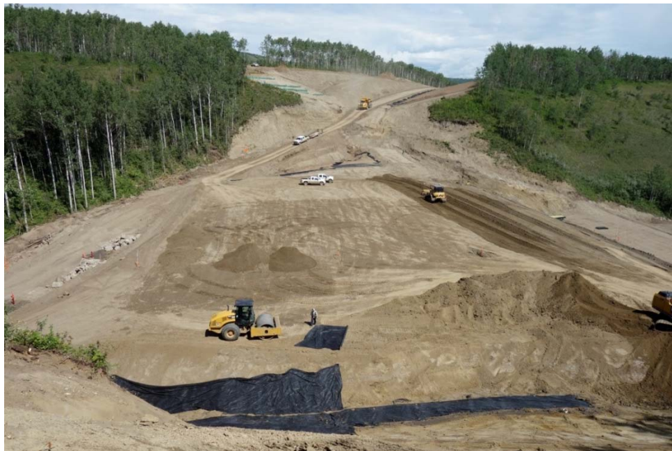
Figure A-4 L3 Gully Fill in Progress (Morgan Construction)
