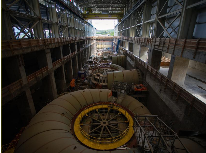
Figure A-7 Powerhouse component installation is underway for Units 1, 2, and 3 (May 2021)
