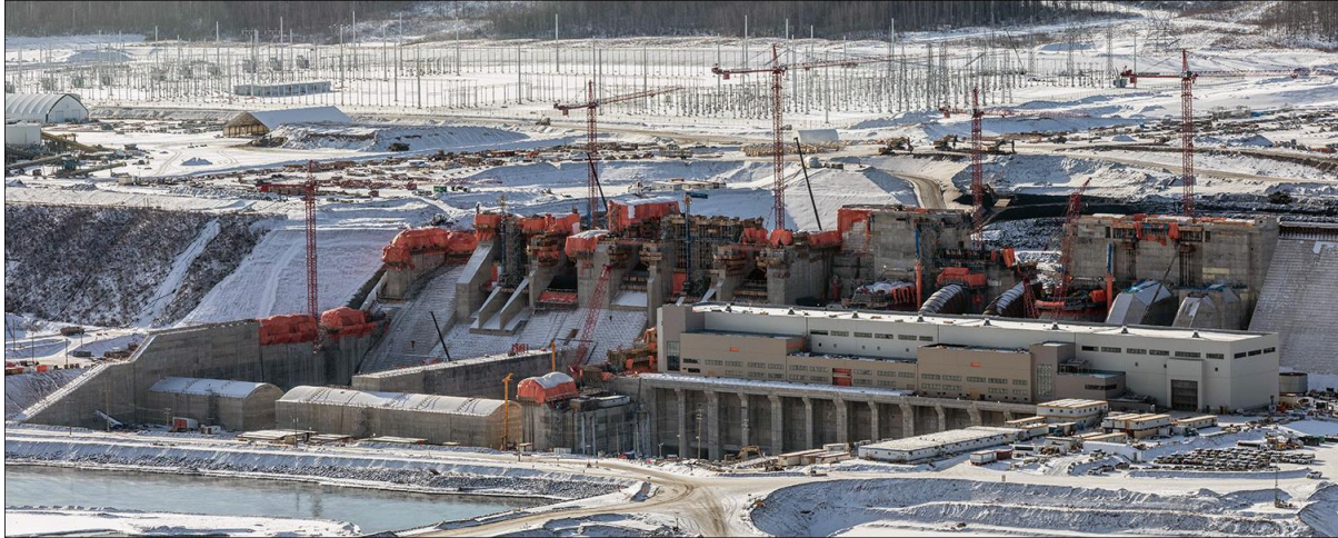
Figure A-1 View of the powerhouse and spillways (January 2022)
