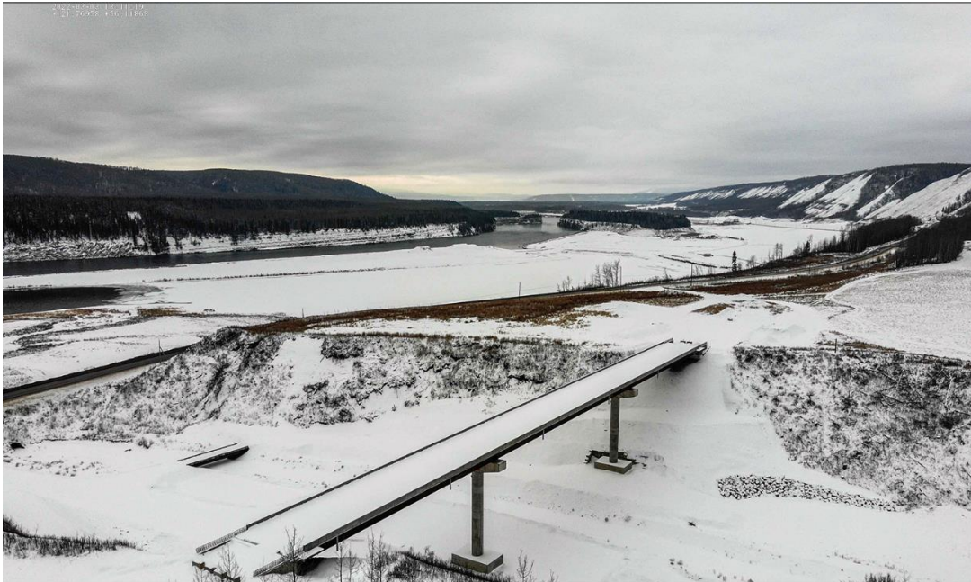
Figure A-10 Dry Creek bridge is complete (March 2022)
