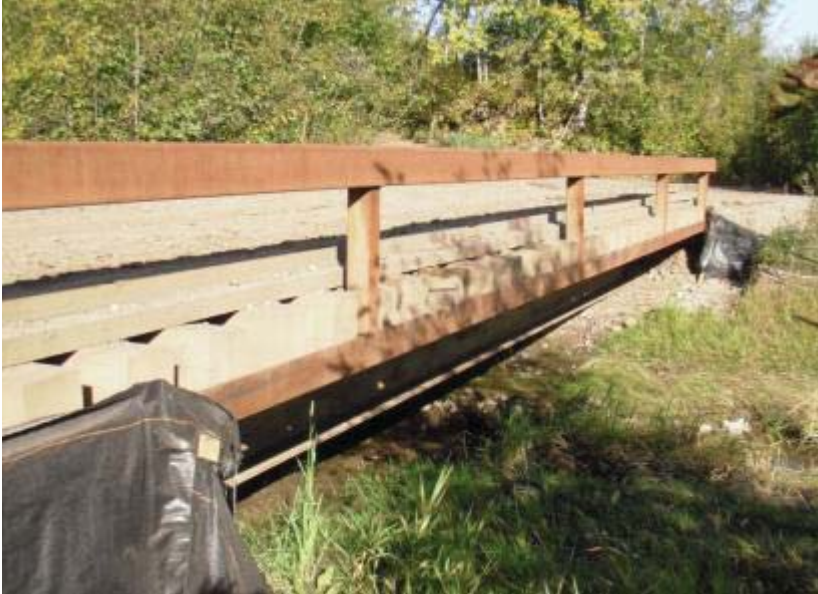
Photograph I-3 Existing abutment bridge Credit: Industrial Forestry Service Ltd. (2011)
