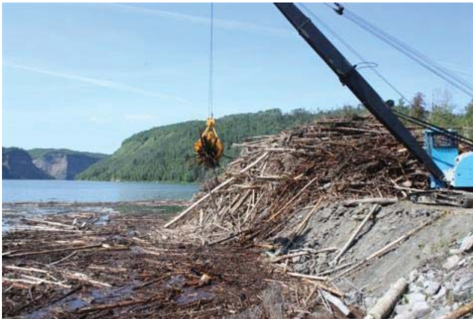
Photograph 10 Crane used to extract woody debris
